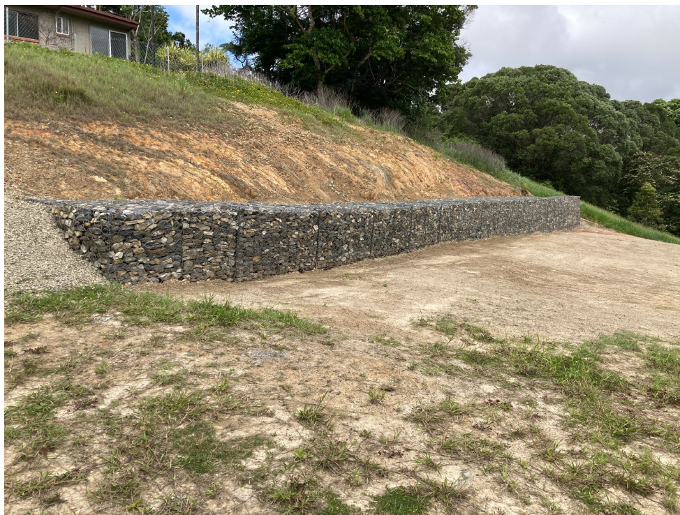
Kuranda Heights Cemetery Gabion Wall
