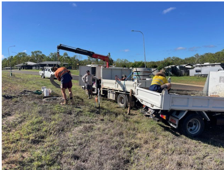
Sewer manhole remediation works
