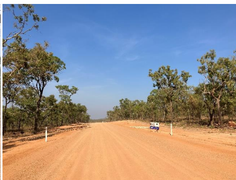
Ootann Road – after (subgrade level)
