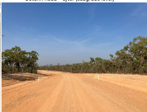
Ootann Road – after (subgrade level)
