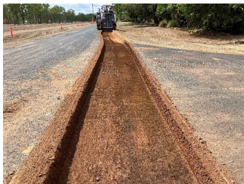
Removing existing failed pavement layer
