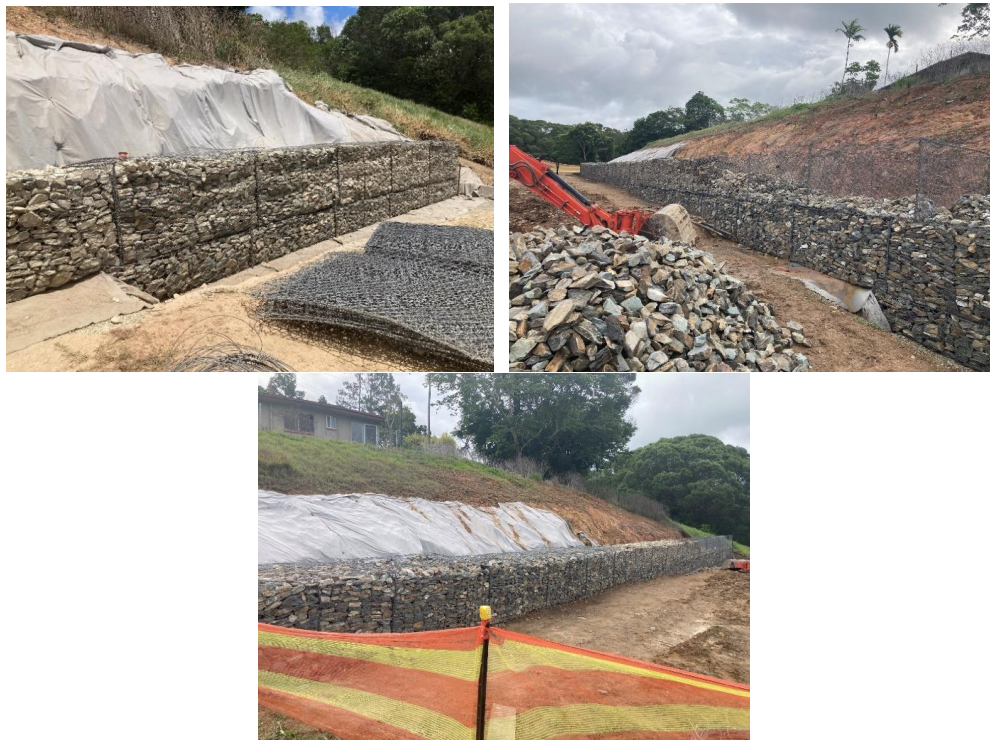
Gabion wall construction continuing
