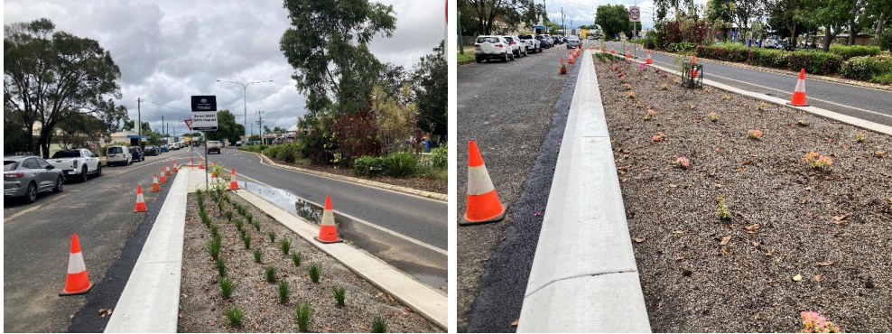
Location 8: Concrete kerbs installed and planting underway on Byrnes Street Median Island on the eastern side of the road between Railway Avenue (northern end) and Granite Creek
