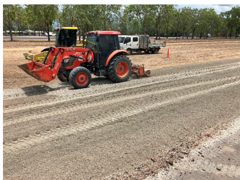
Blending bagged cement into base layer
