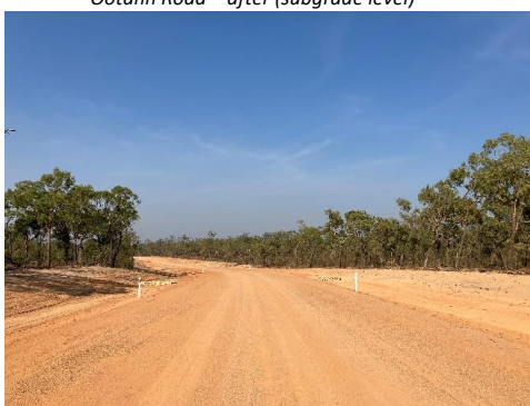
Ootann Road – after (subgrade level)
