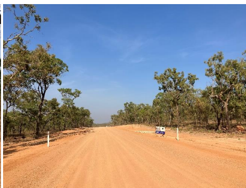
Ootann Road – after (subgrade level)
