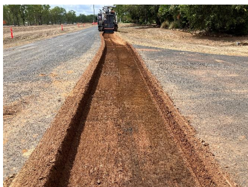
Removing existing failed pavement layer
