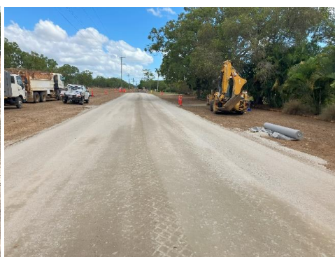
Completed base pavement layer
