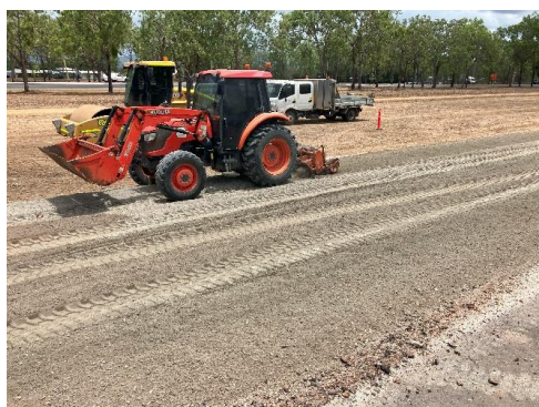
Blending bagged cement into base layer
