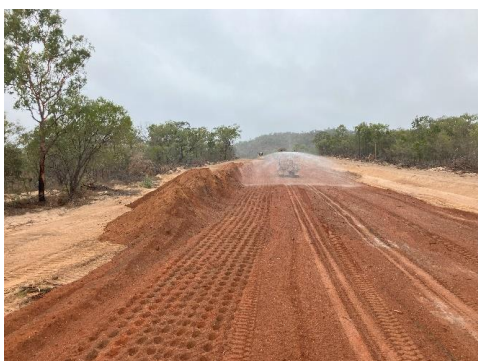
Embankment filling operation
