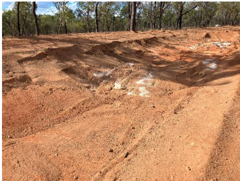
Exposed rock in table drains
