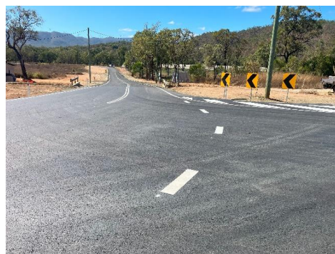
Channel overflow crossing – after
