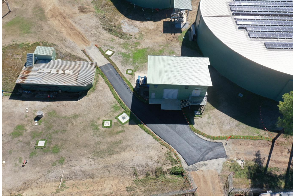
Site works have now been completed
