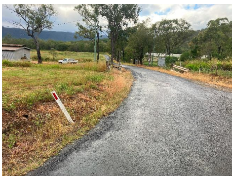
Channel overflow crossing - before
