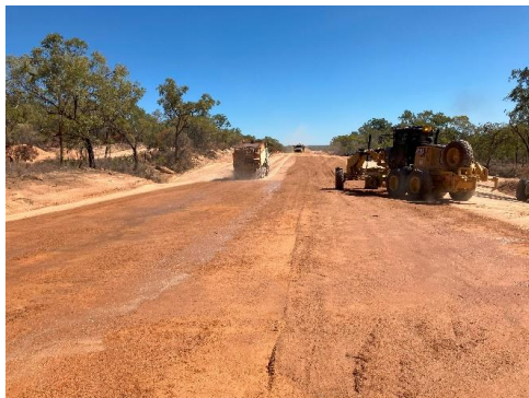
Earthworks to subgrade level
