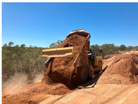
Cut to fill works
