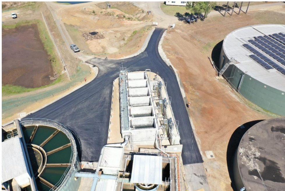
Installation and reinstatement of road pavement
