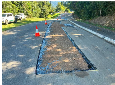
Milled section prepped for asphalt
