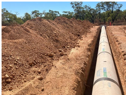
New RCP Culvert 13H
