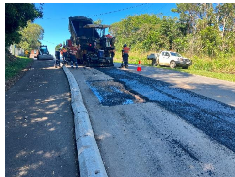
Asphalt density testing
