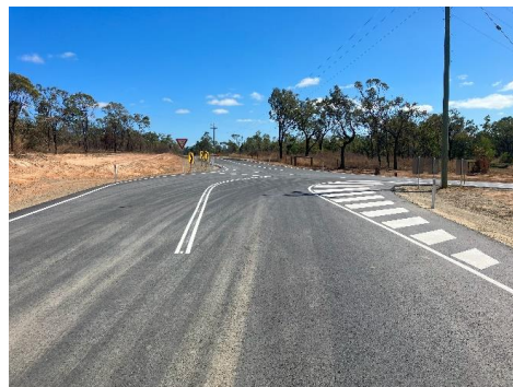
Collins Weir Road/Springmount Road Intersection - after
