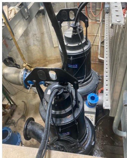
Installation of new valving and installation of new infrastructure.
