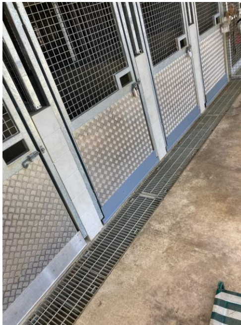
Mareeba Animal Refuge repairs
