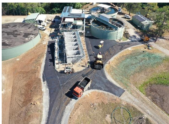
Installation and reinstatement of road pavement
