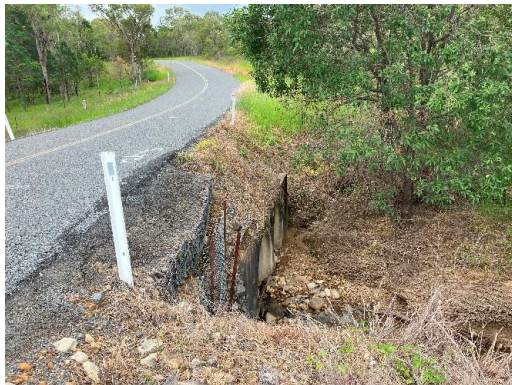
Culvert D – Before
