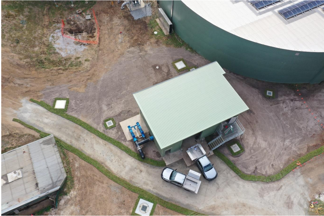
Site works generally have now been completed.
