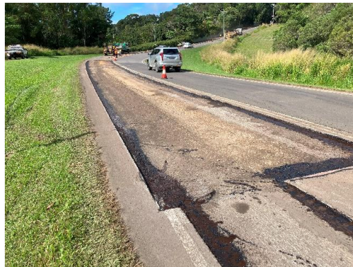
Milled section prepped for asphalt
