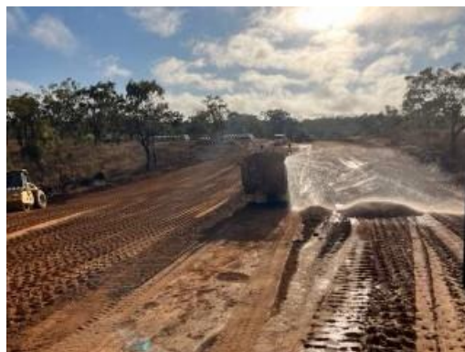
Earthworks to subgrade level
