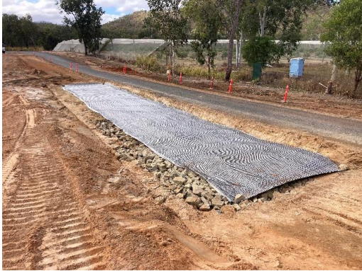
Treating failed subgrade section
