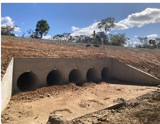
Culvert B - After
