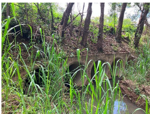
Culvert B - Before
