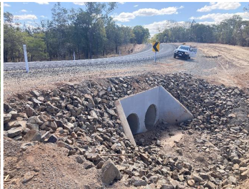
Culvert D - After
