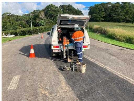
Asphalt density testing
