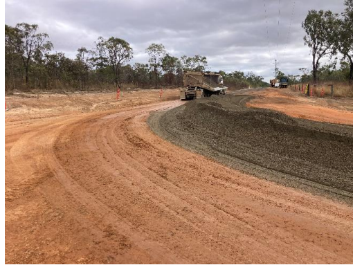
Importing subbase layer
