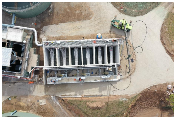
Installation of inlet troughs and electrical and mechanical equipment under way
