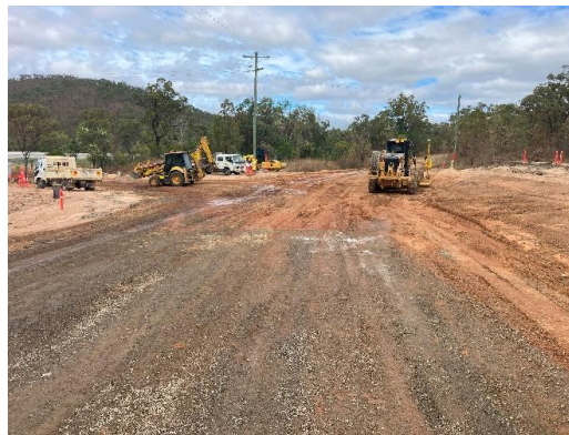
Collins weir Road intersection earthworks
