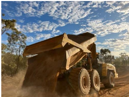
Cut to fill operations
