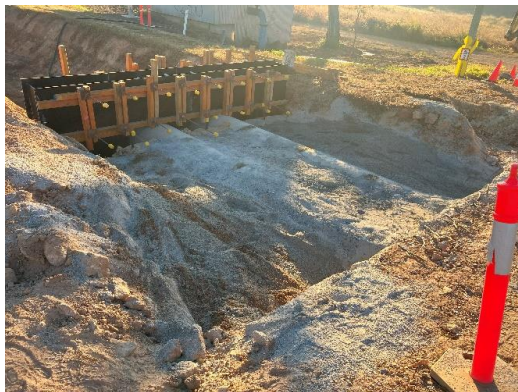
Widening existing channel overflow crossing
