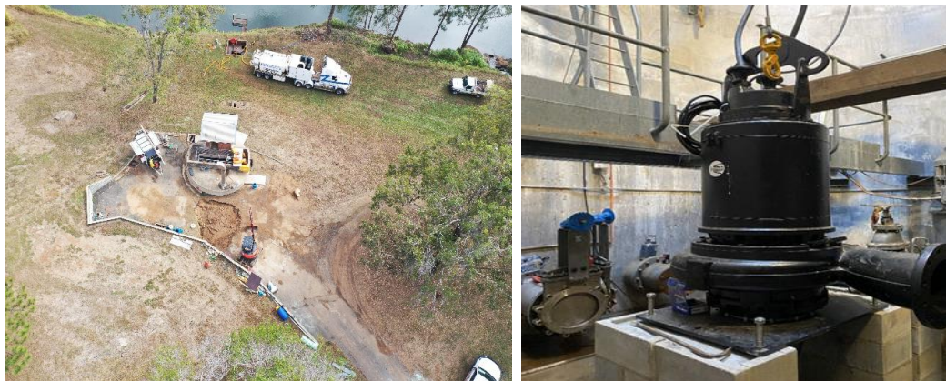
Installation of new valving and installation of new infrastructure.
