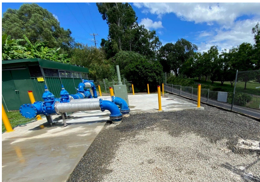
Photo 3 Granite Creek Sewerage Pump Station Refurbishment
