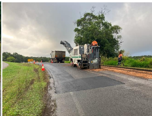
Milling of failed section
