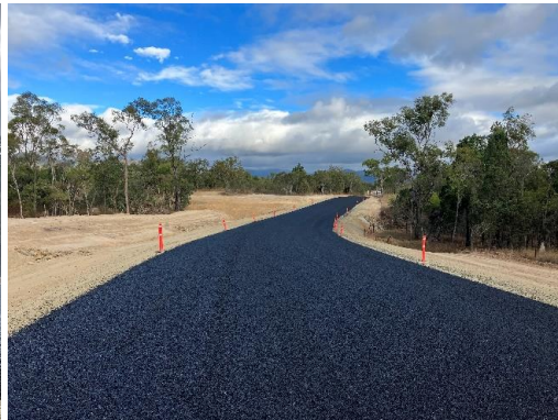
Section 1 seal complete
