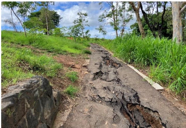
Granite Creek Asphalt Path – 08/01/2024
