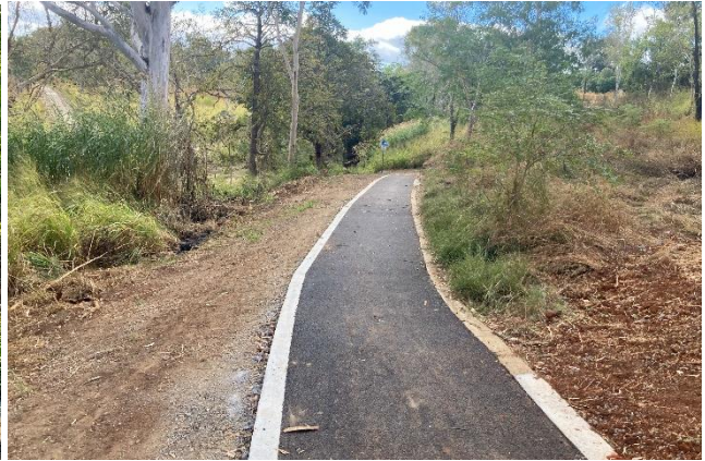
Granite Creek Asphalt path – 26/06/2024
