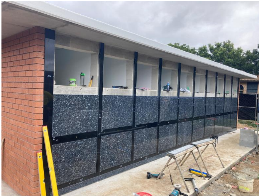
Mareeba Cemetery Mausoleum Wall Construction Nearing Completion
