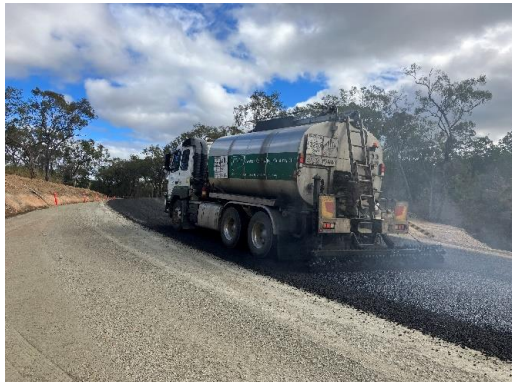
Application of bitumen prior to 10mm second coat
