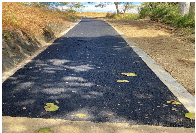
Granite Creek Asphalt path – 26/06/2024
