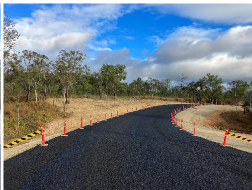
Section 3 seal complete
