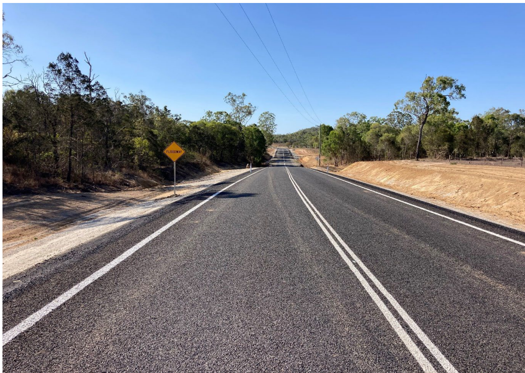
Photo 4 R2R Bilwon Road Rehabilitation and Culverts
