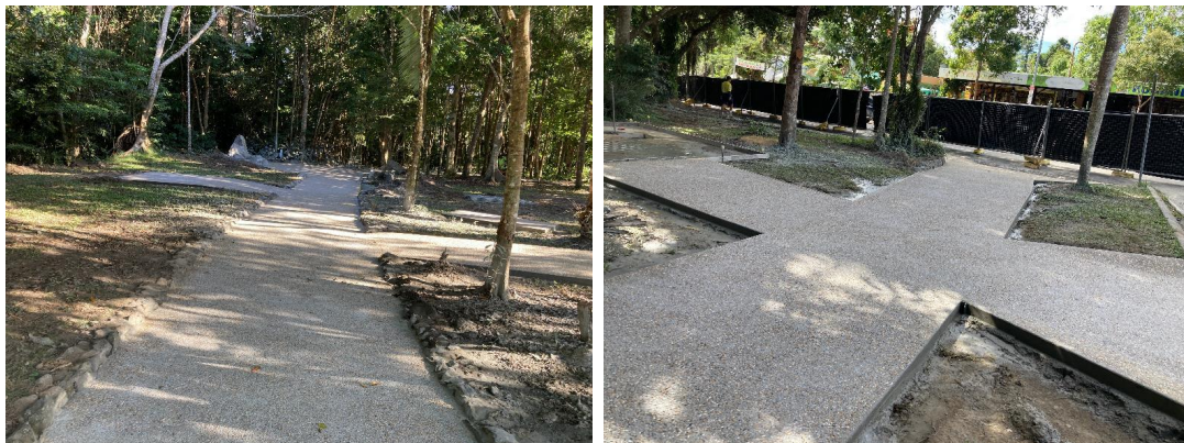
Upgrade footpaths and picnic setting slabs
