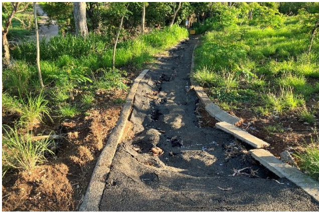
Granite Creek Asphalt Path – 08/01/2024
