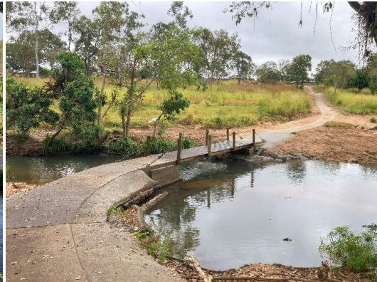
Pedestrian bridge after repair
