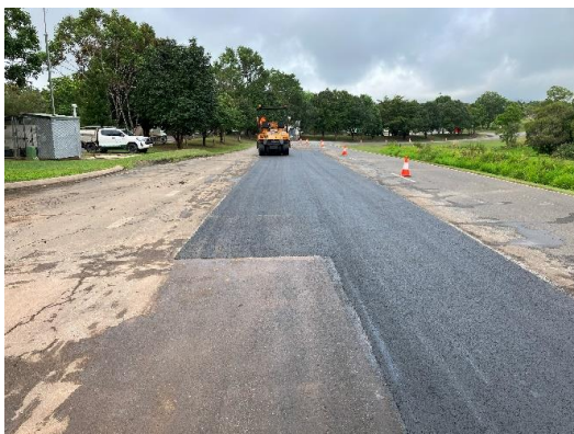
Compaction of asphalt filling
