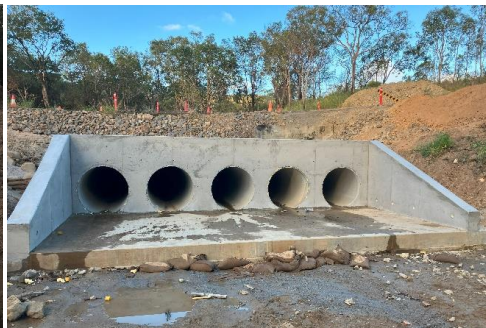
Culvert B completed
