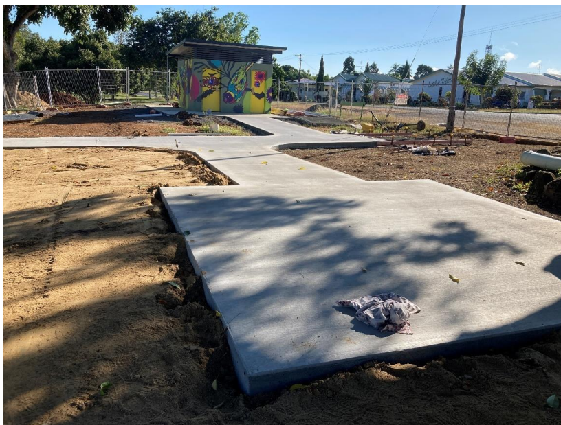
Bicentennial Lakes Mason Street New Public Toilet, footpaths and picnic shelter pad construction
