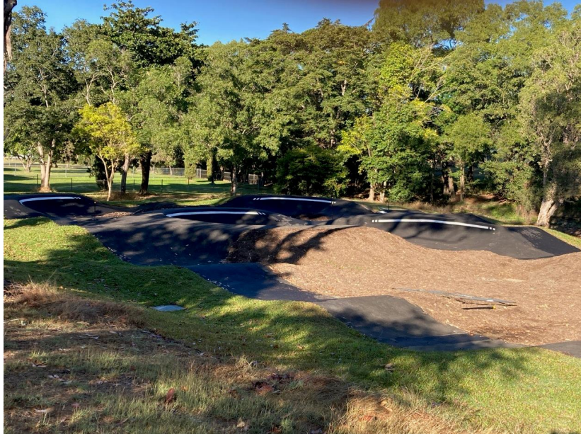
Bicentennial Lakes Mason Street Pump Track Construction
