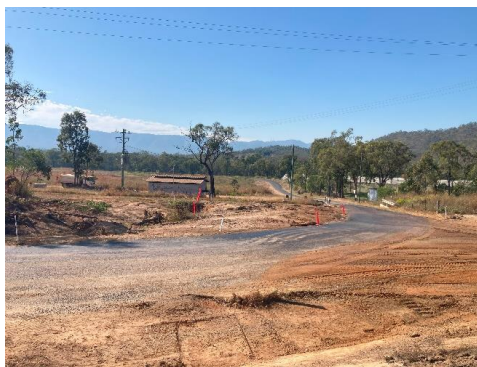
Intersection set out
