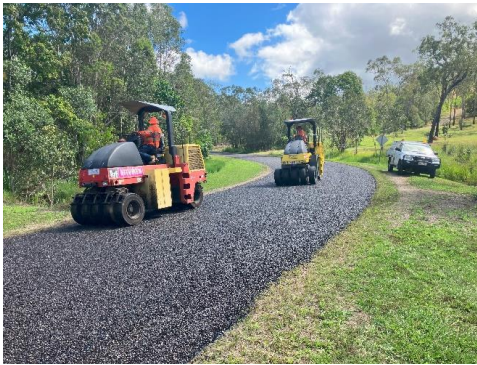
McLeans Bridge Road
