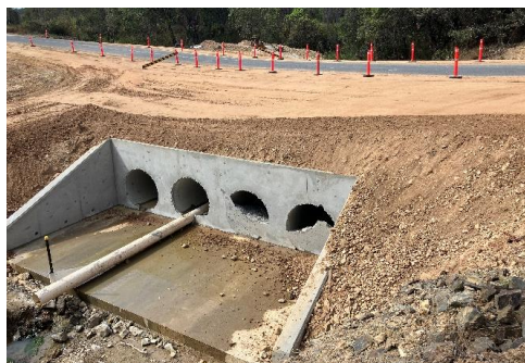
Culvert C1-C2 completed
