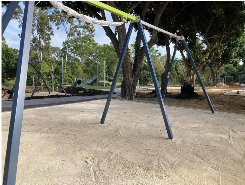
Bicentennial Lakes Mason Street Playground Construction – Swing
