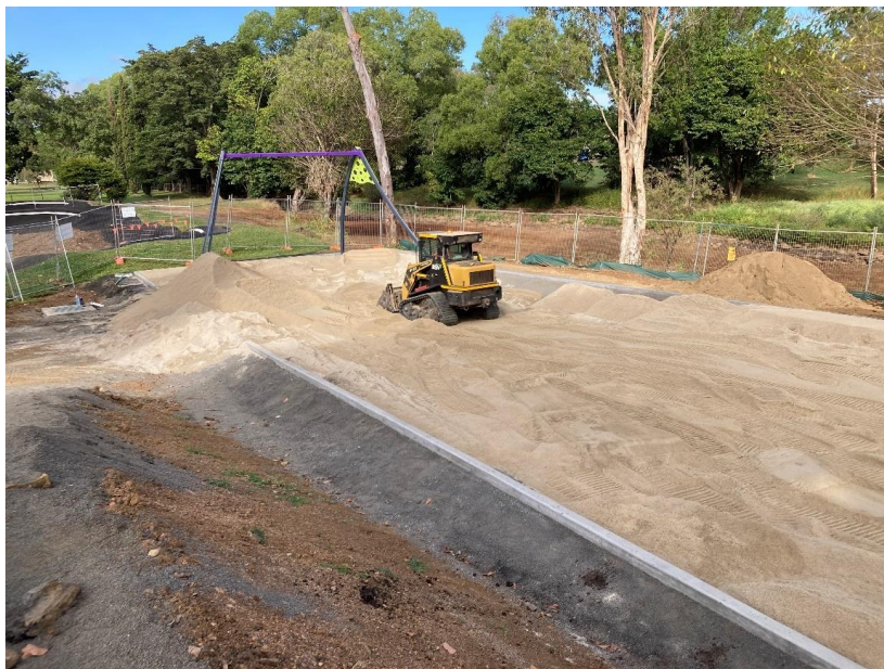
Bicentennial Lakes Mason Street Playground Construction – Flying Fox
