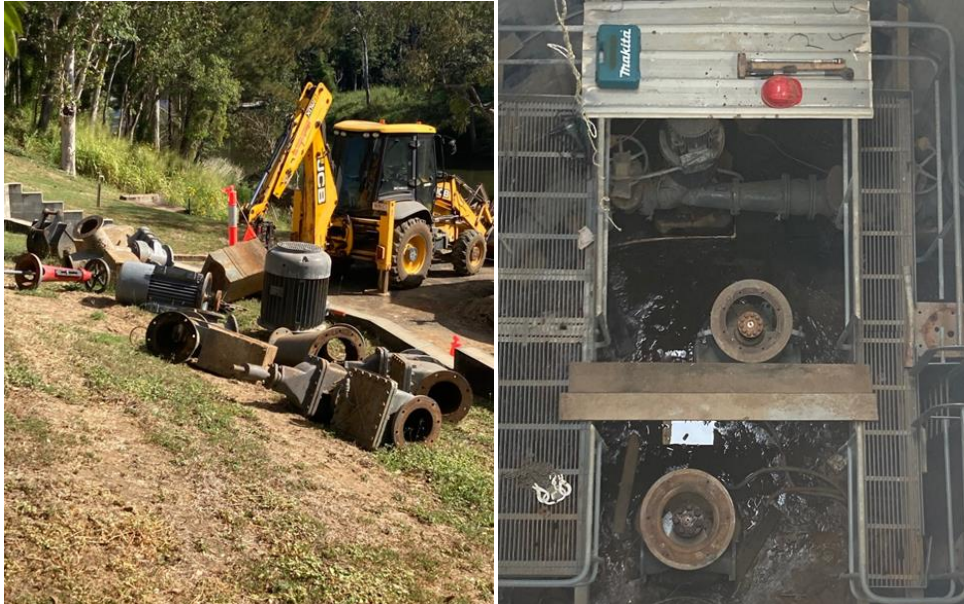
Civil Stripping out the old pumps and pipe work to make way for new infrastructure.
