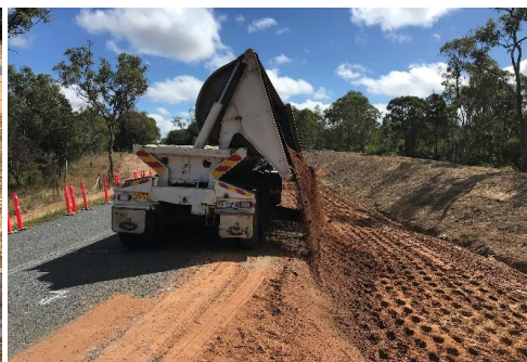
Commencement of earthworks
