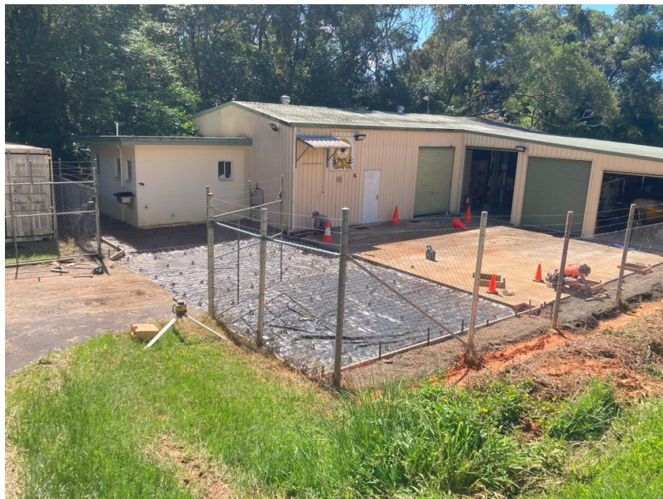
Kuranda SES Facility – Concrete Slab Construction
