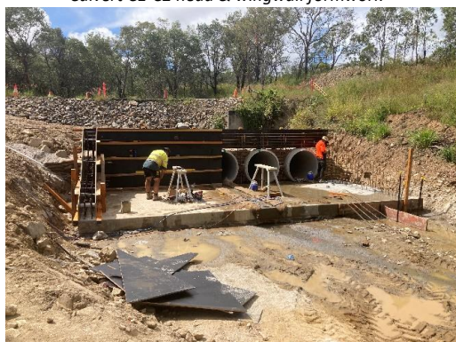
Culvert B head & wingwall formwork
