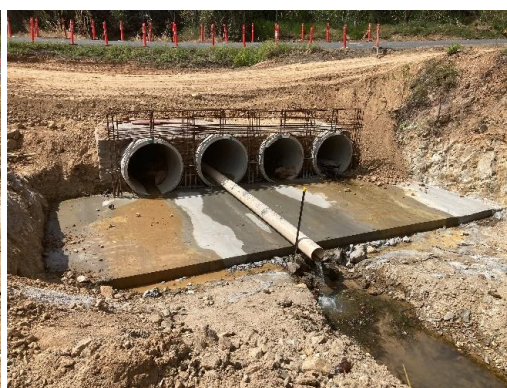
Culvert C1-C2 after apron installation
