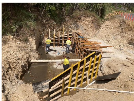
Culvert C1-C2 head & wingwall formwork
