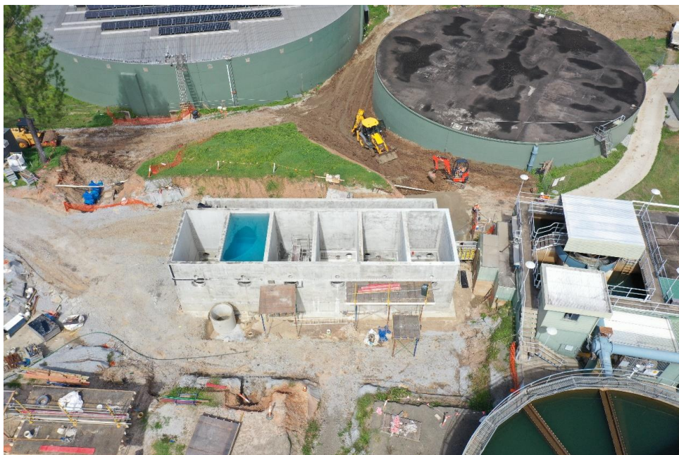
Concrete construction of new filter cell modules and installation of new pipe work
