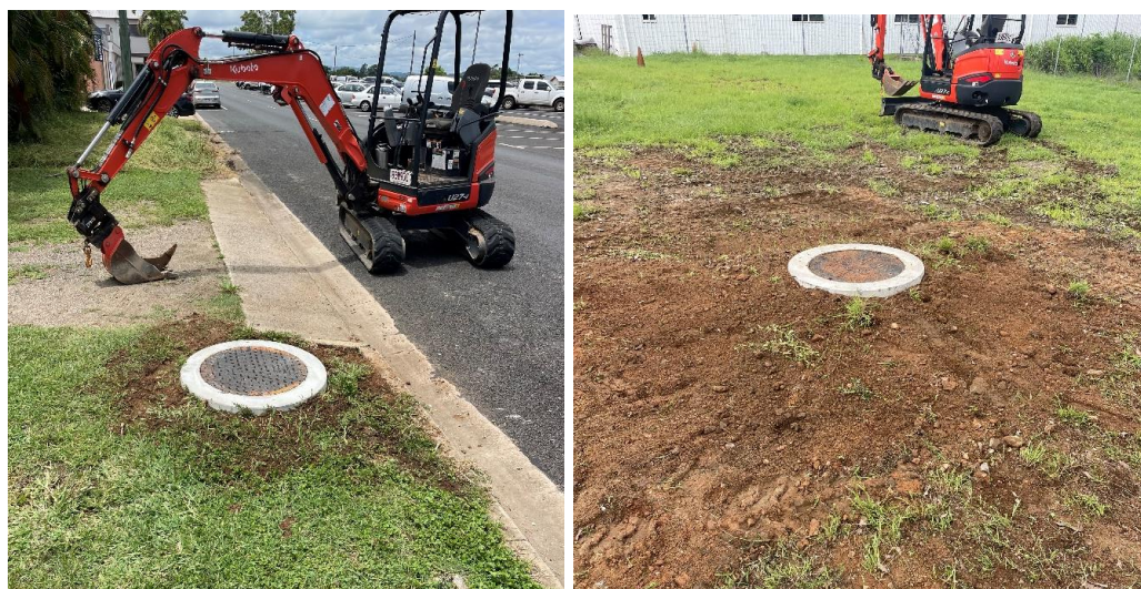
Sewer manhole remediation works
