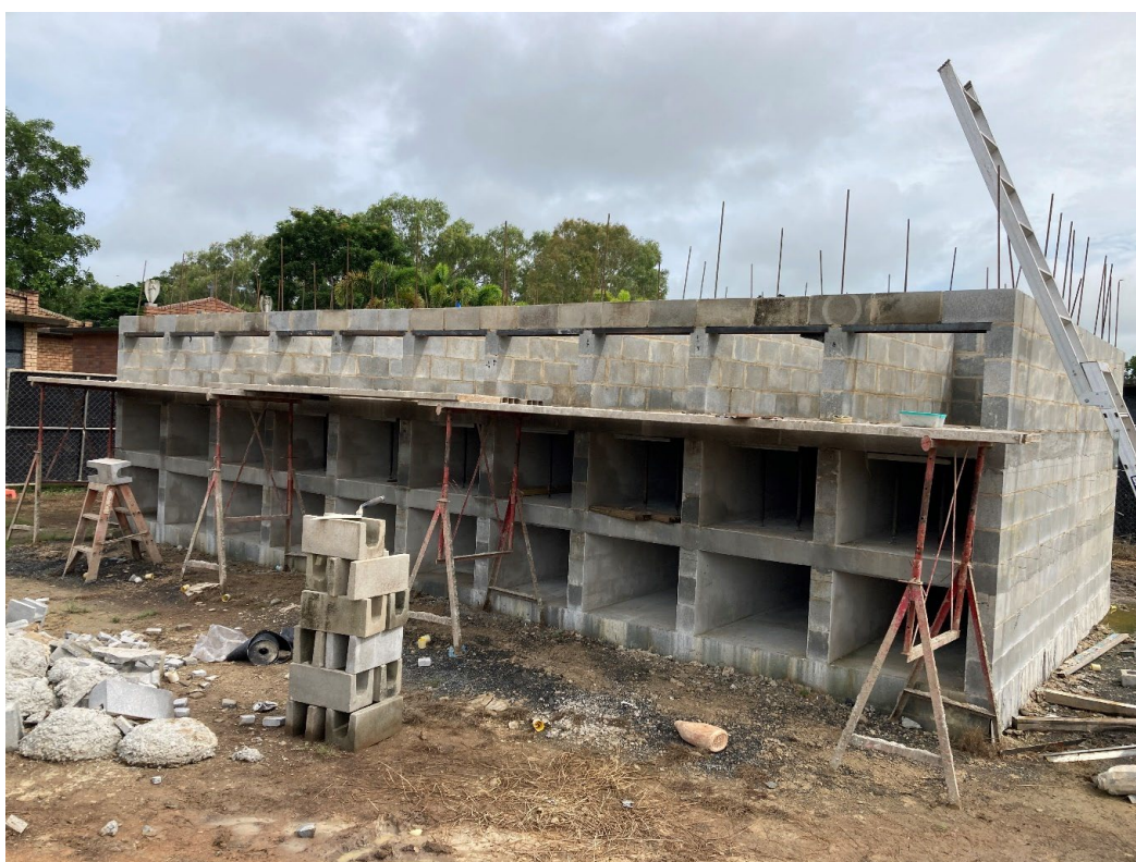
Mausoleum Wall Construction
