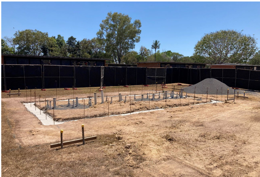
Mausoleum Wall Footings Construction
