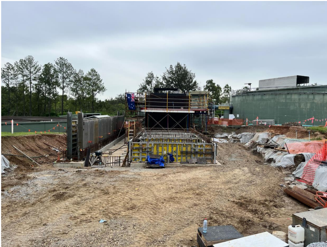
Concrete construction of new filter cell modules.
