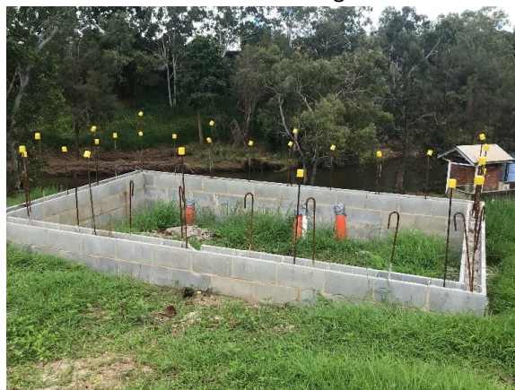
Electrical cabling conduits installed
