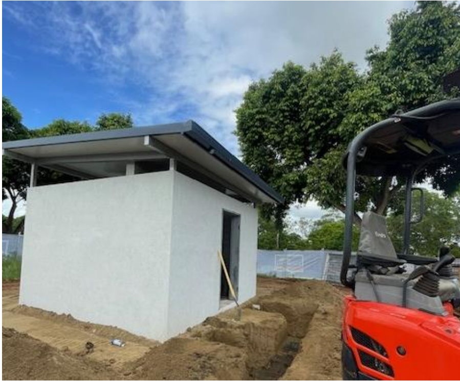
Bicentennial Lakes Southern Section New Public Toilet Construction
