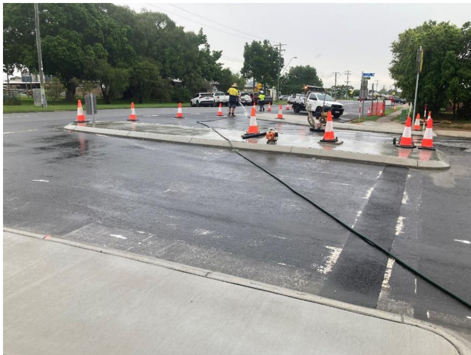
Concrete island infill
