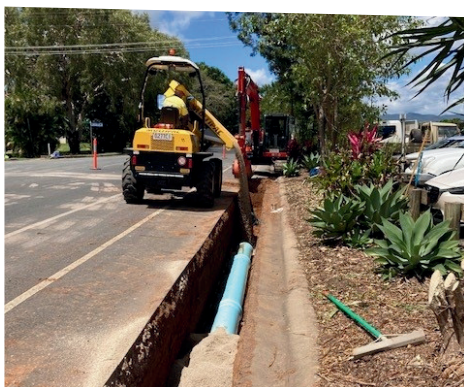
AC water main replacement program
