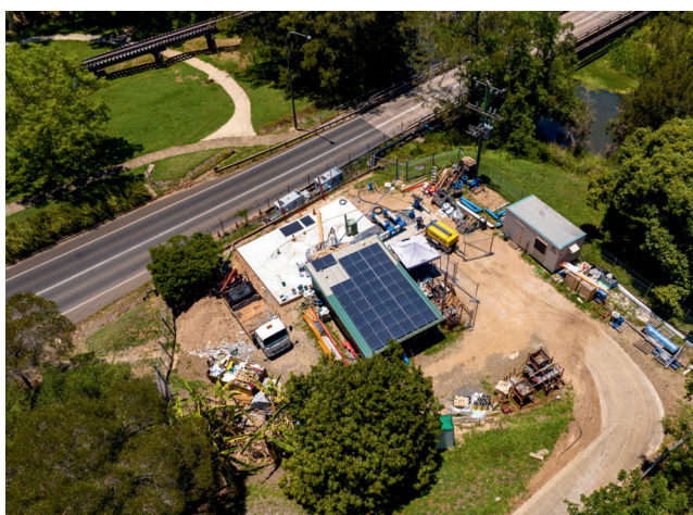
Granite Creek Pump Station upgrade, 2022
