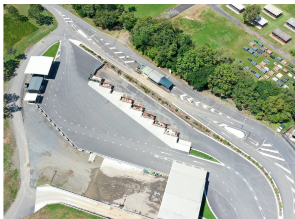
Mareeba Transfer Station Redevelopment, 2021
