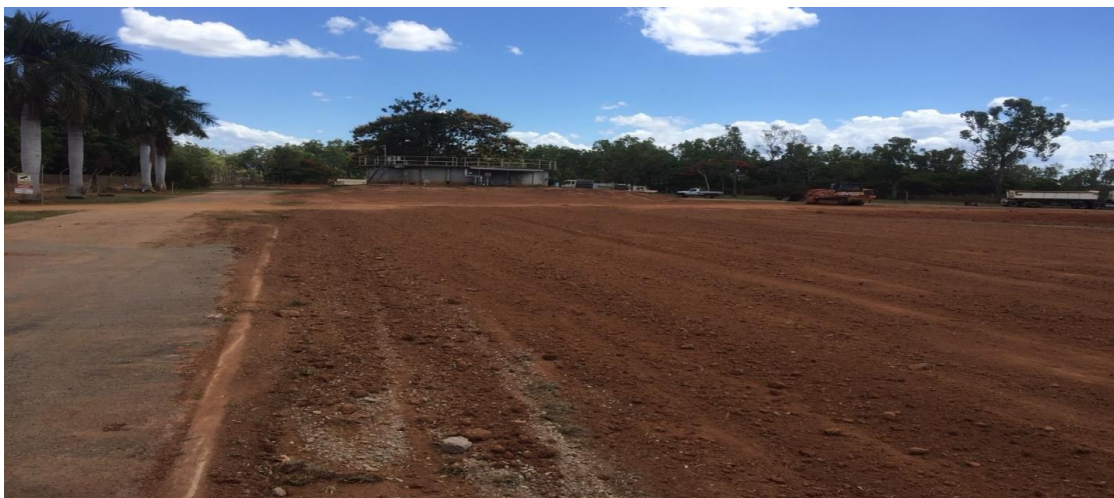
Site reinstatement following demolition of old Mareeba Wastewater Treatment Plant
