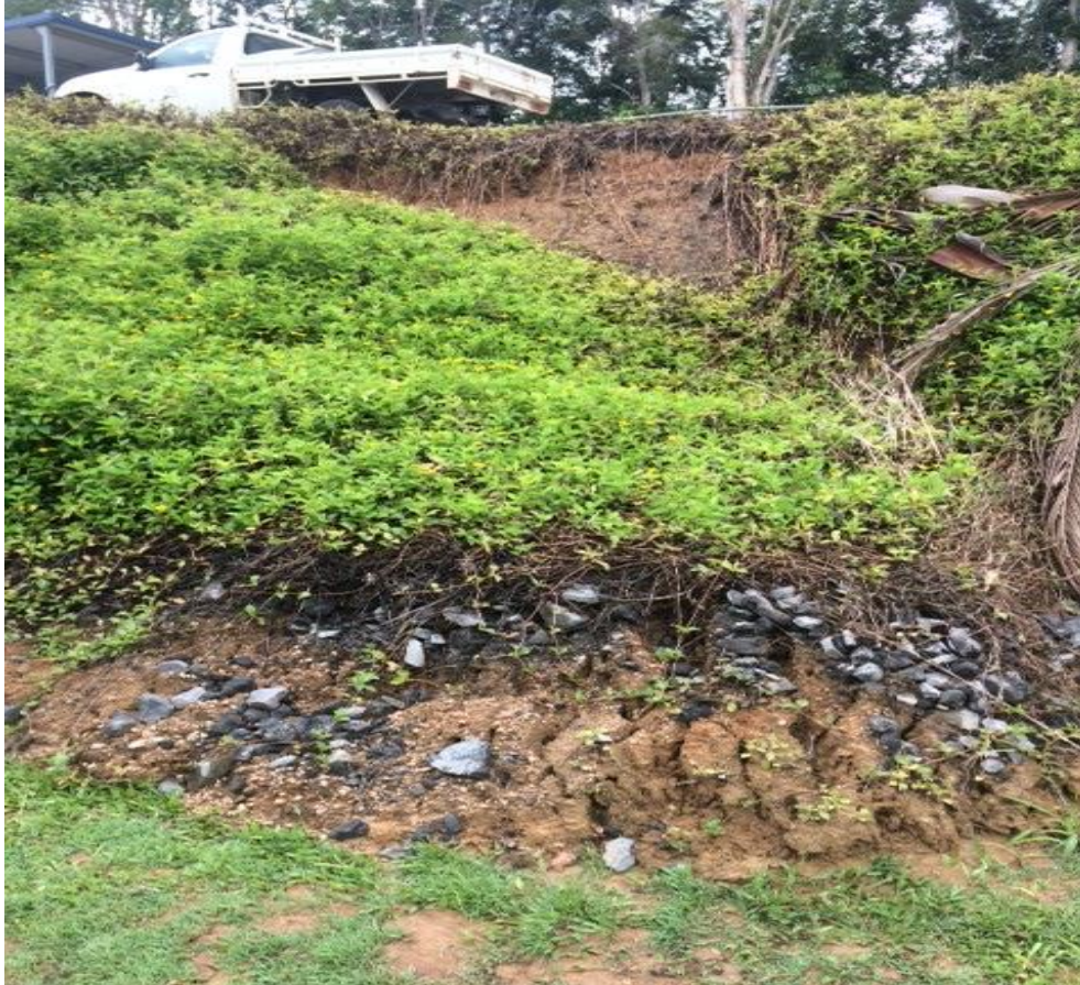
Kuranda WWTP embankment slip
