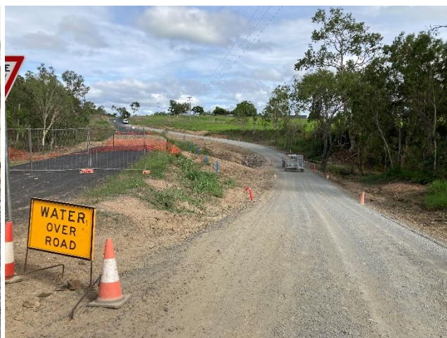
Temporary Side track and causeway – Emerald End Road
