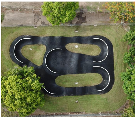
Dimbulah Pump Track Practical Completion
