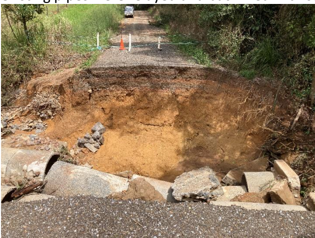
Collapsed RCP culvert – Black Mountain Road, Julatten
