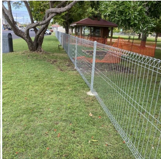
Dimbulah Railway Park and Pump Track Fence Construction
