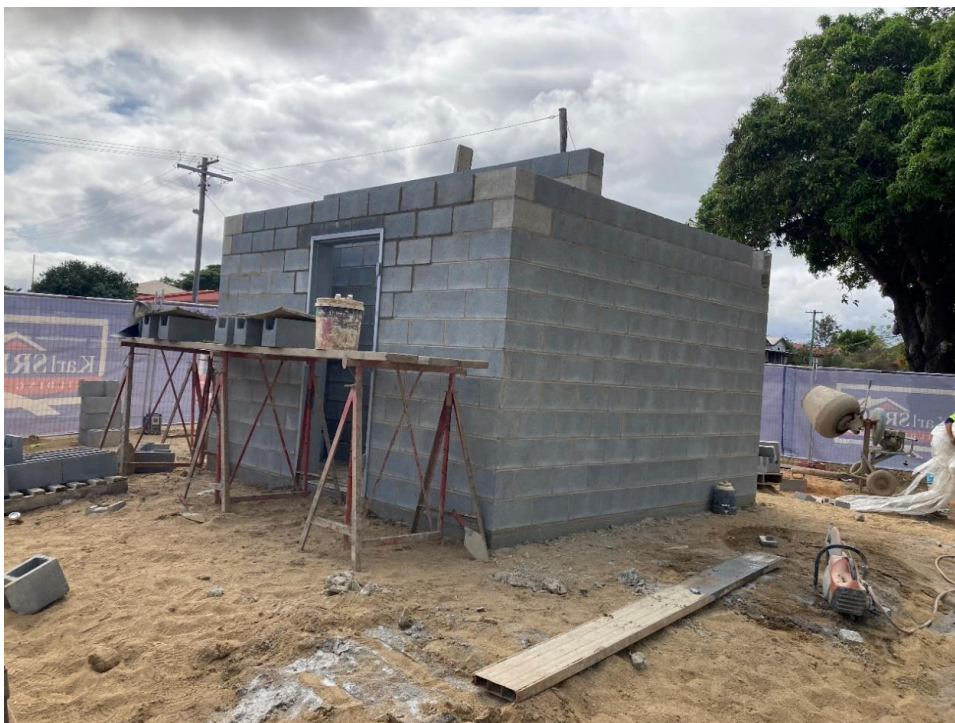
Bicentennial Lakes Toilet Amenities Block Construction
