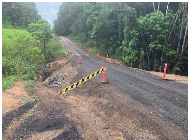
Temporarily repaired RCP culvert – Black Mountain Road, Julatten
