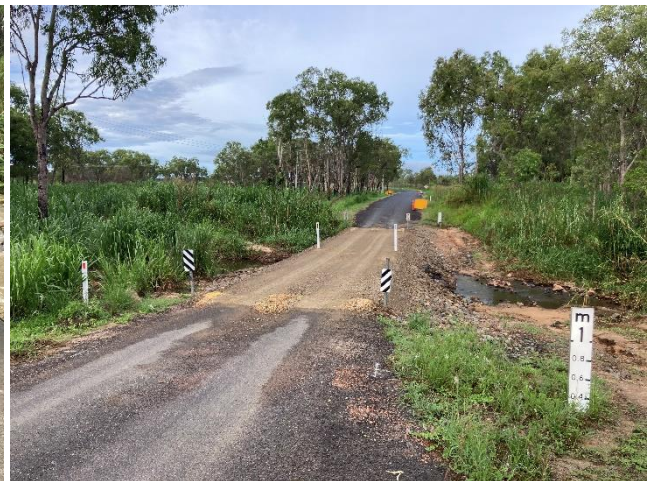
Temporarily repaired causeway – Carman Road
