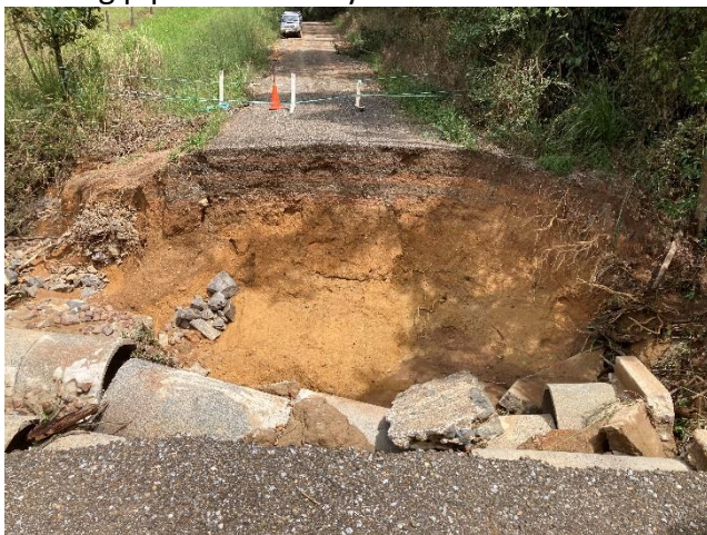
Collapsed RCP culvert – Black Mountain Road, Julatten
