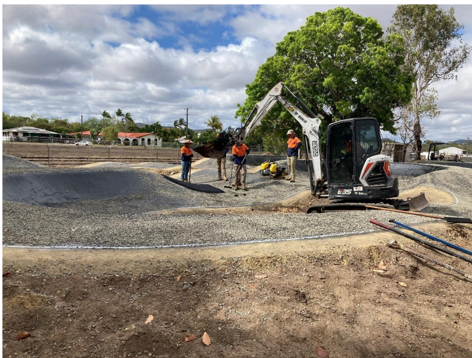
Dimbulah Pump Track Asphaltting Works Commencement
