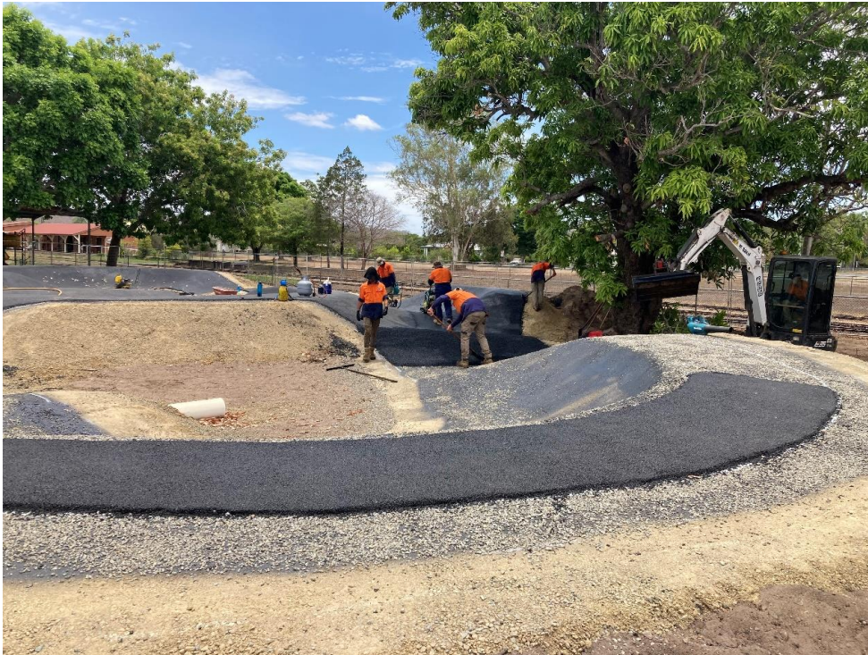
Dimbulah Pump Track Asphalting Works Commencement
