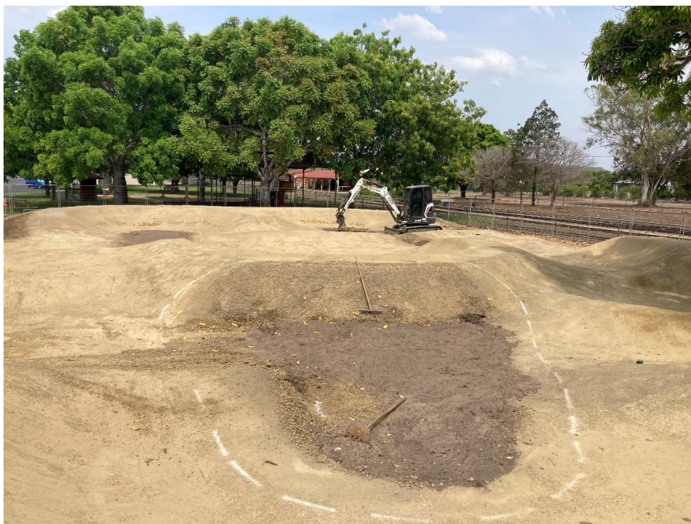
Dimbulah Pump Track Shaping Earthworks
