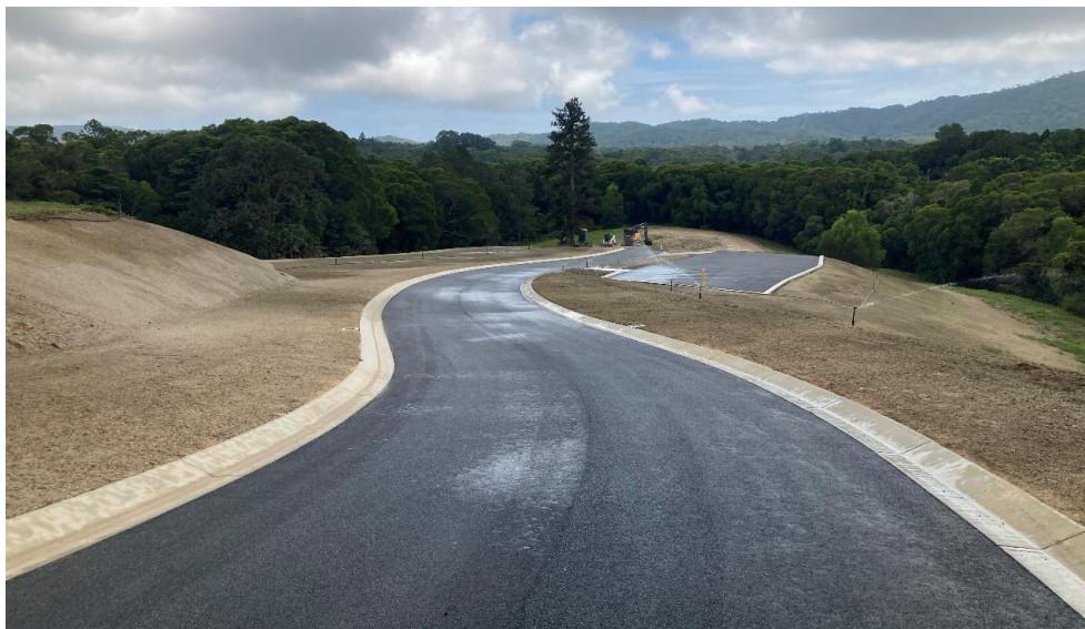
Kuranda Heights Cemetery – new road works complete
