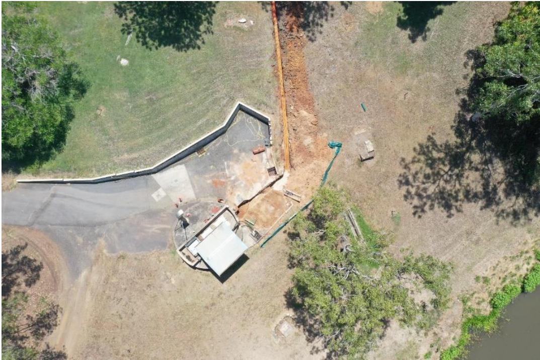
Civil earthworks continuing along with raw water pump shed construction
