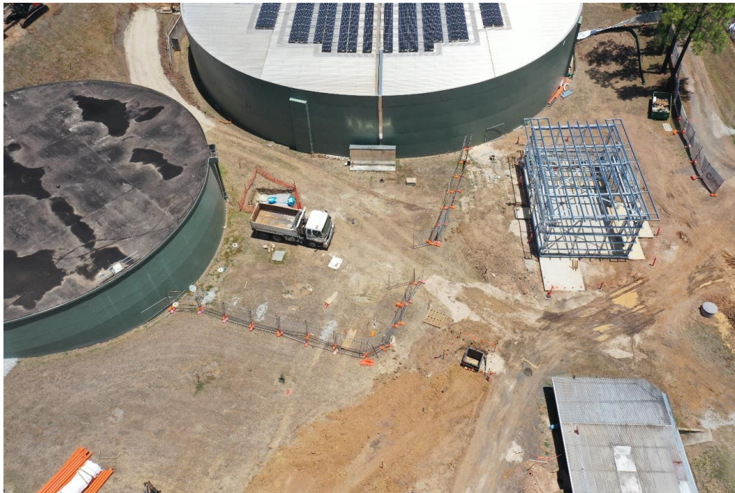
Civil earthworks continuing along with pump shed construction
