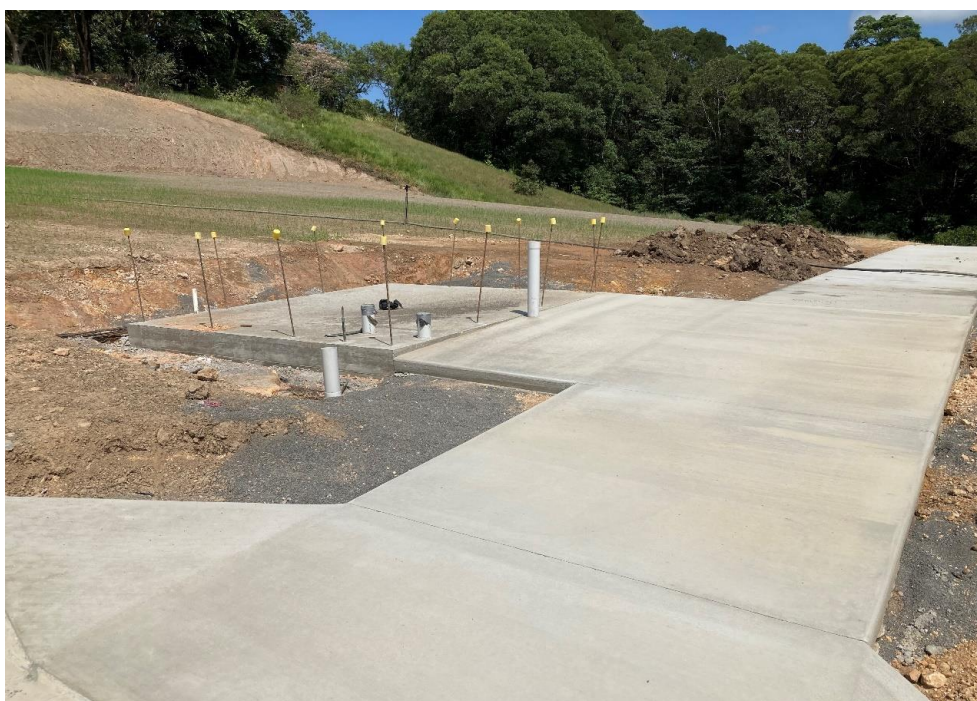
Kuranda Heights Cemetery – New footpath complete and toilet construction commenced.
