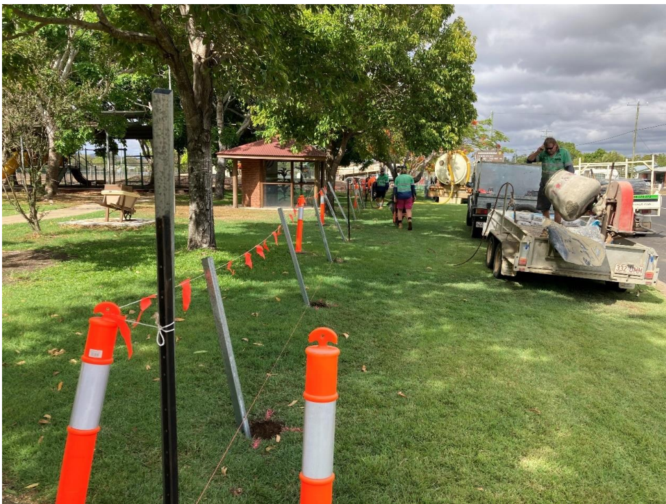
Fence Construction Commencement
