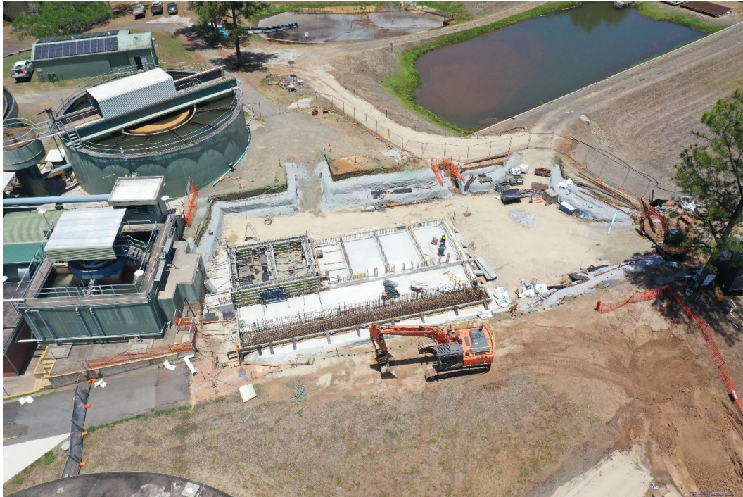
Construction of filtration modules progressing along with civil earthworks
