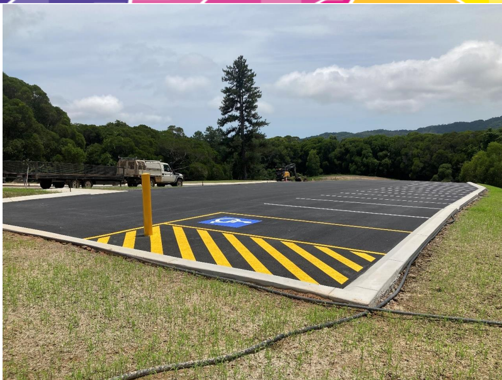
Kuranda Heights Cemetery – new carpark complete
