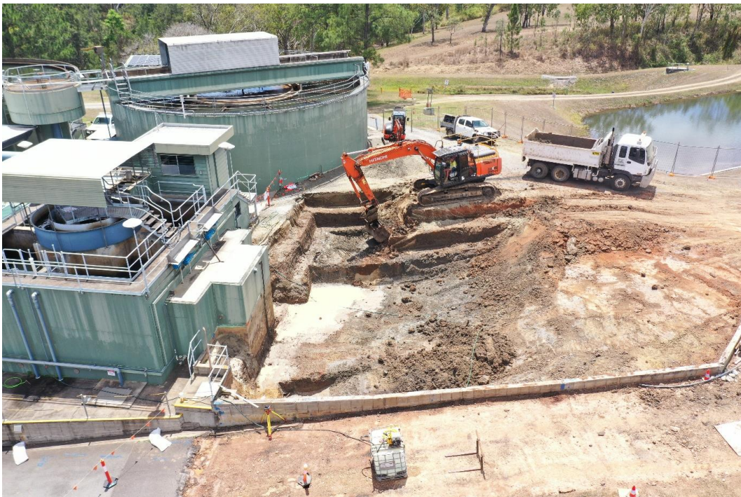
Civil earthworks for new filtration system
