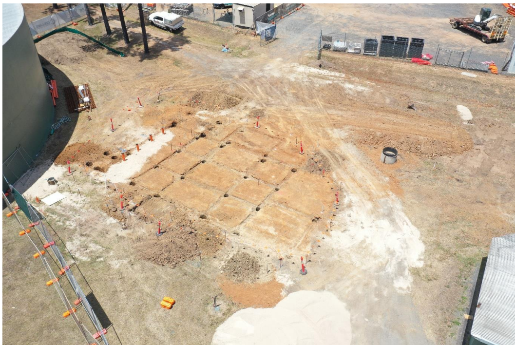
Civil earthworks for booster station
