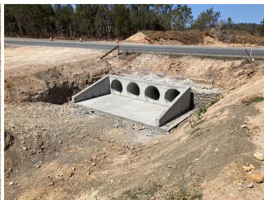
Completed culvert and apron
