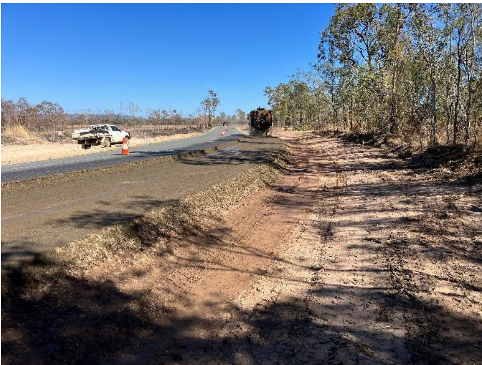
Replacing milled shoulder with road base
