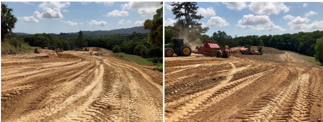
Bulk Earthworks to shape surface profile
