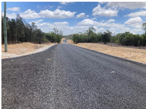
Completed two coat seal
