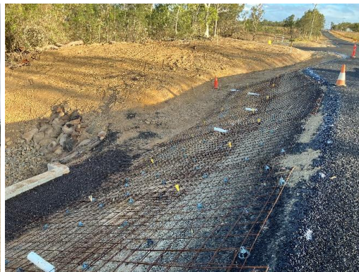
Concrete batter protection reinforcing
