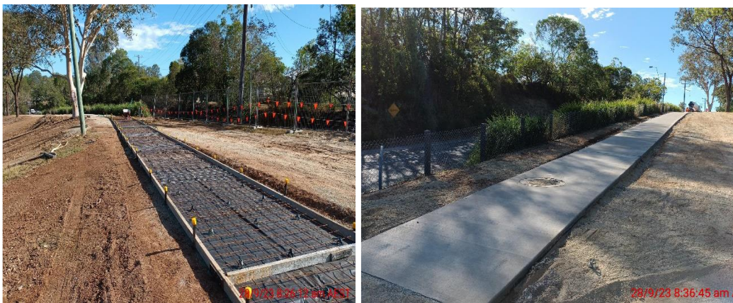
Reinstatement of concrete footpath through Rotary Park
