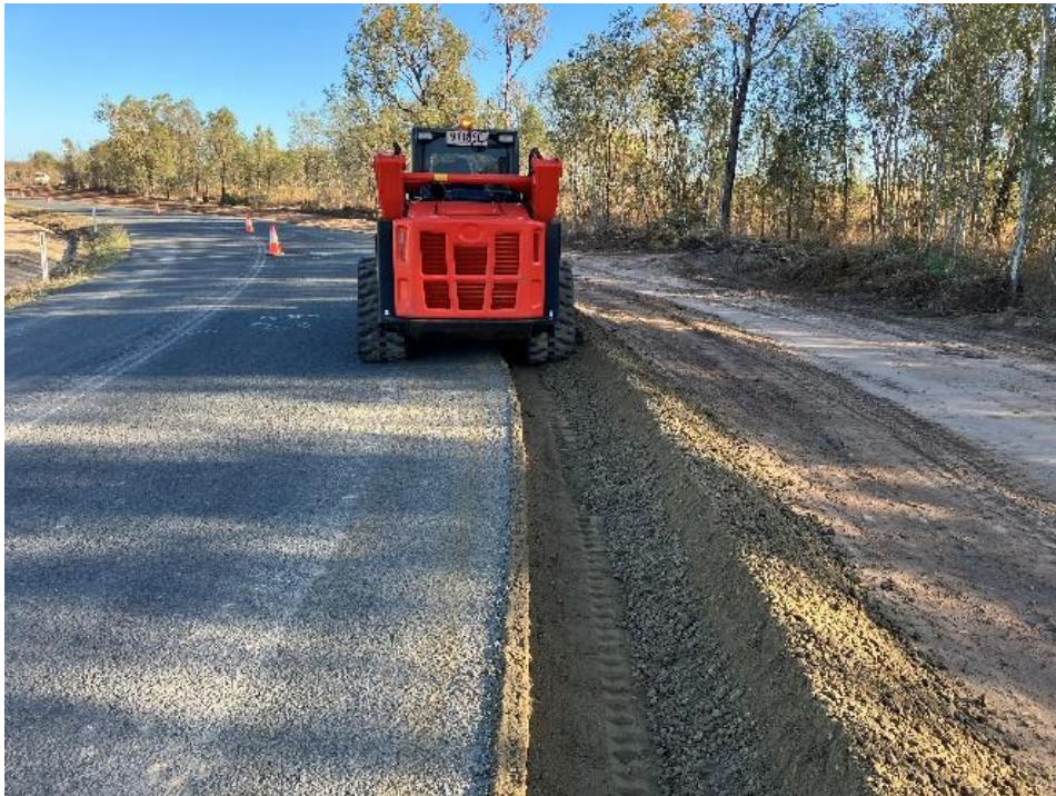
Milling out existing shoulder
