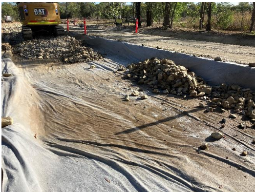
Unsuitable material replacement
