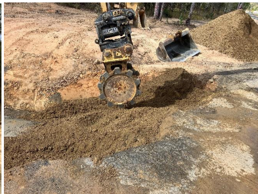
Pipe overlay zone compaction
