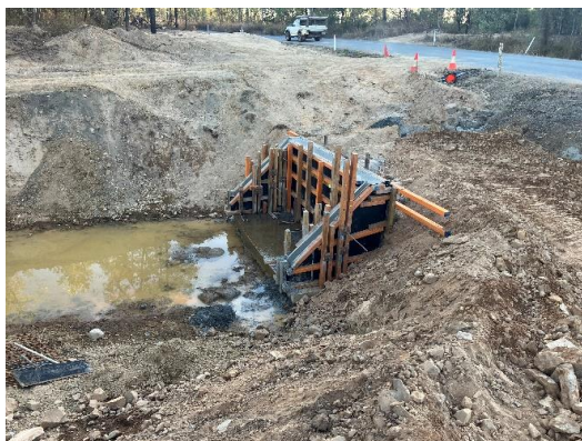
Culvert headwall and apron construction
