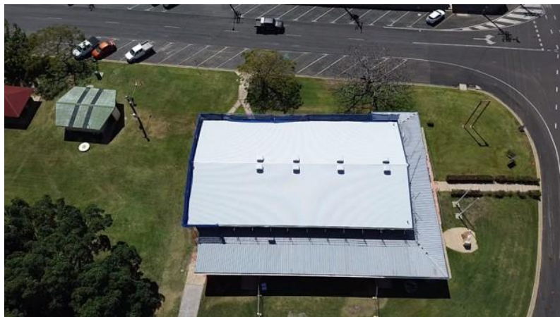
Dimbulah Memorial Hall Roof Replacement and Insulation Upgrade – Project Completion Aerial View
