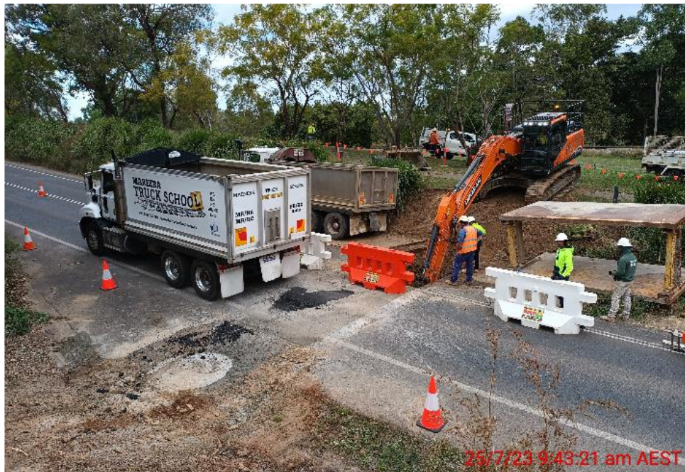
Trenching through Byrnes Street (TMR Corridor) under single lane closure
