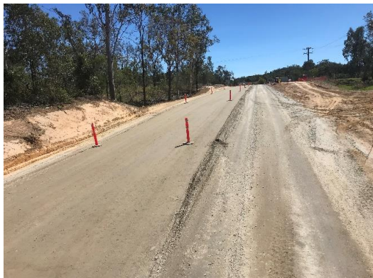
LHS Base layer complete
