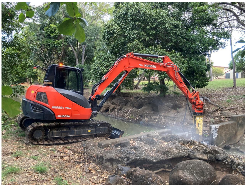
Bicentennial Lakes Southern Section Weir Removal
