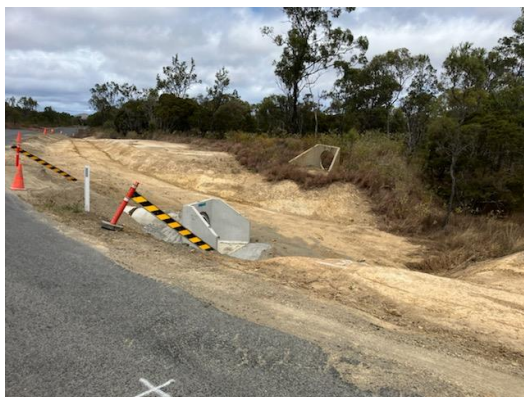
Installed pre-fabricated headwall
