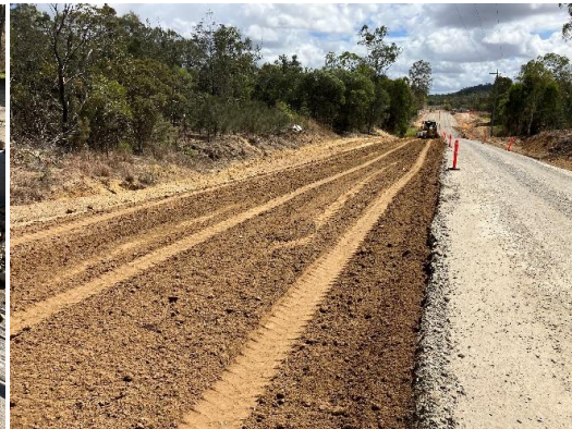
Subbase layer installation
