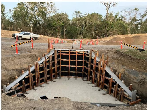
1800Ø RCP headwall after pouring
