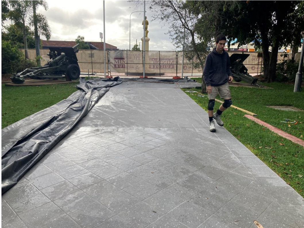
Anzac Park Footpath Replacement – tiling continues
