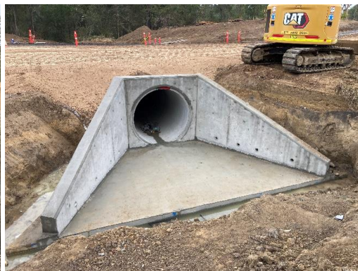
1800Ø RCP headwall complete
