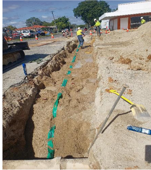
DN300 valve assembly prepped for thrust block concrete pour, and water main marker tape above reinstated DN100 DICL pipe
