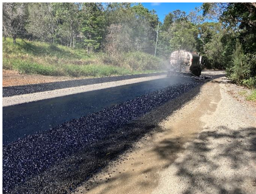
Second coat 10mm seal
