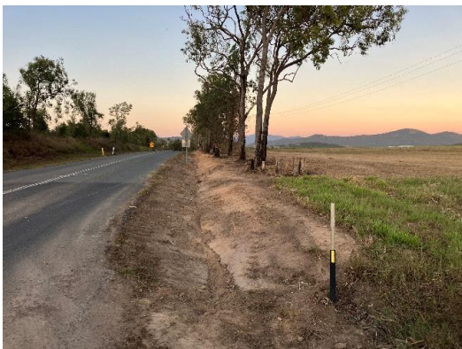
Drainage work – RHS
