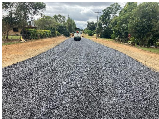
10mm aggregate bitumen seal over full width
