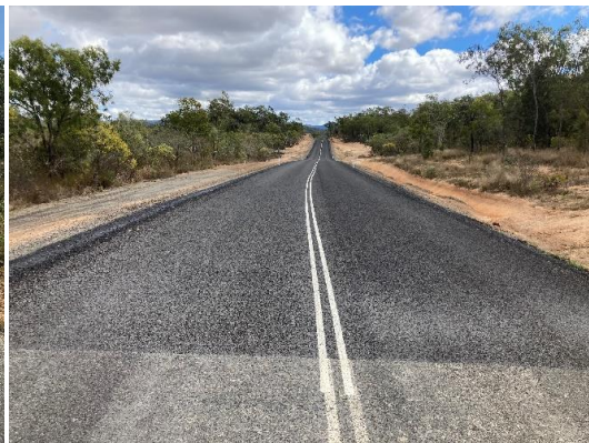
Wolfram Road after
