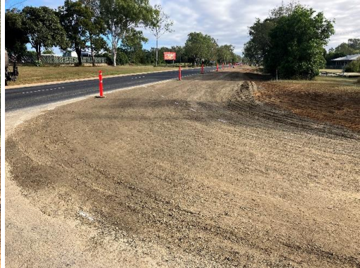
Replaced shoulder material
