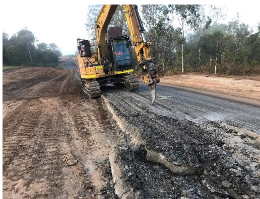
Excavate to new subgrade design
