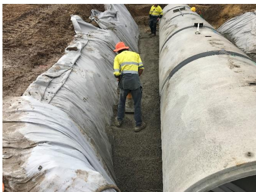
Culvert haunch zone treatment
