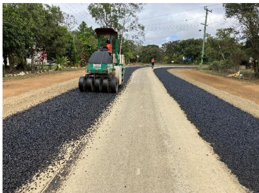
16mm aggregate bitumen seal
