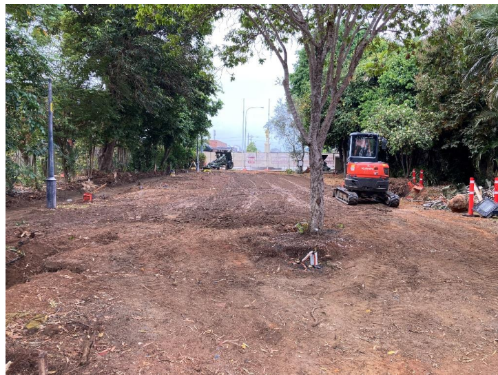
Anzac Park Mareeba Construction Works
