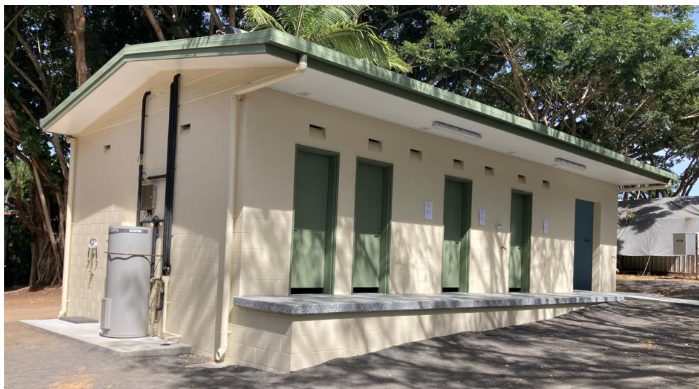
Riverside Caravan Park Amenities block western elevation
