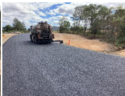
Second coat bitumen sealing
