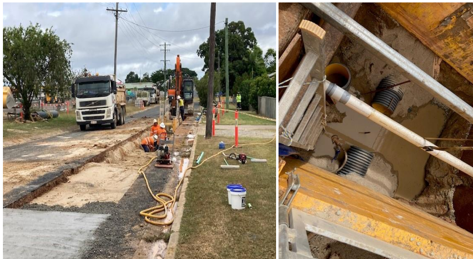
Strattmann Street installation of the new 450mm diameter gravity sewer main
