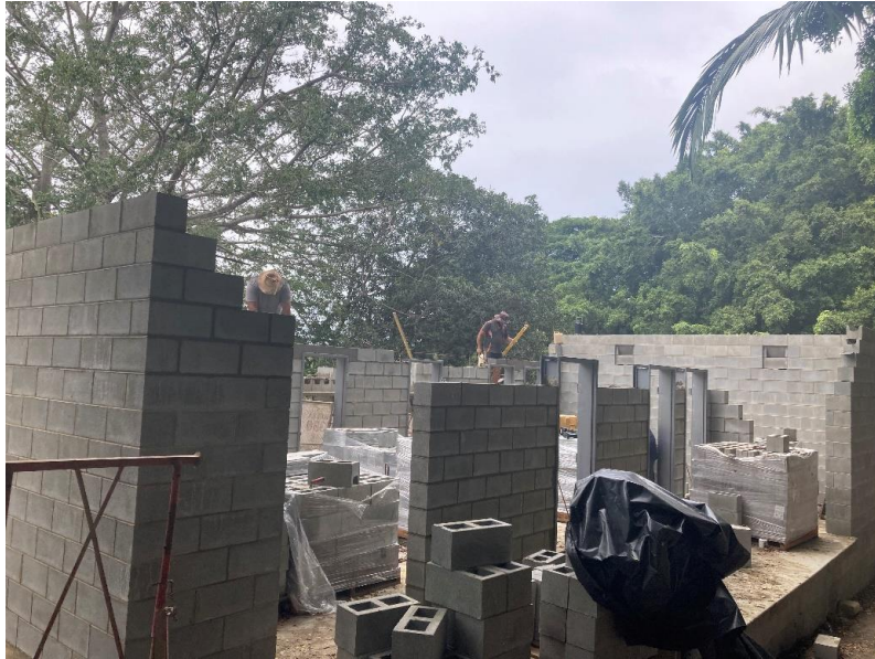
Riverside Caravan Park Amenities Construction
