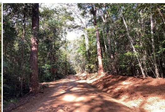
Bump Track Gravel Re-Sheet
