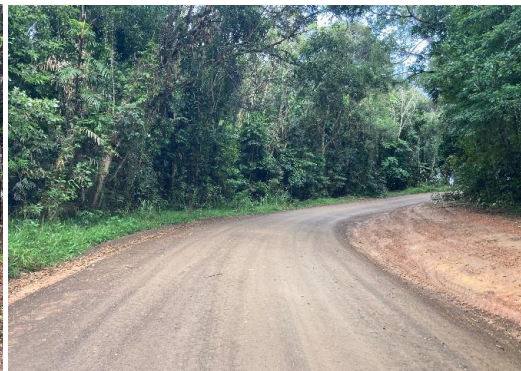
Black Mountain Road Gravel Re-Sheet
