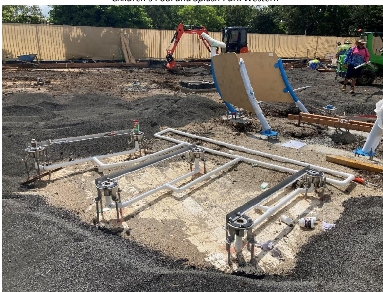
Plumbing and Play Equipment Preparation
