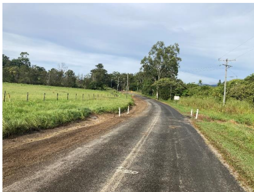
Euluma Creek Road Drain Reestablishment
