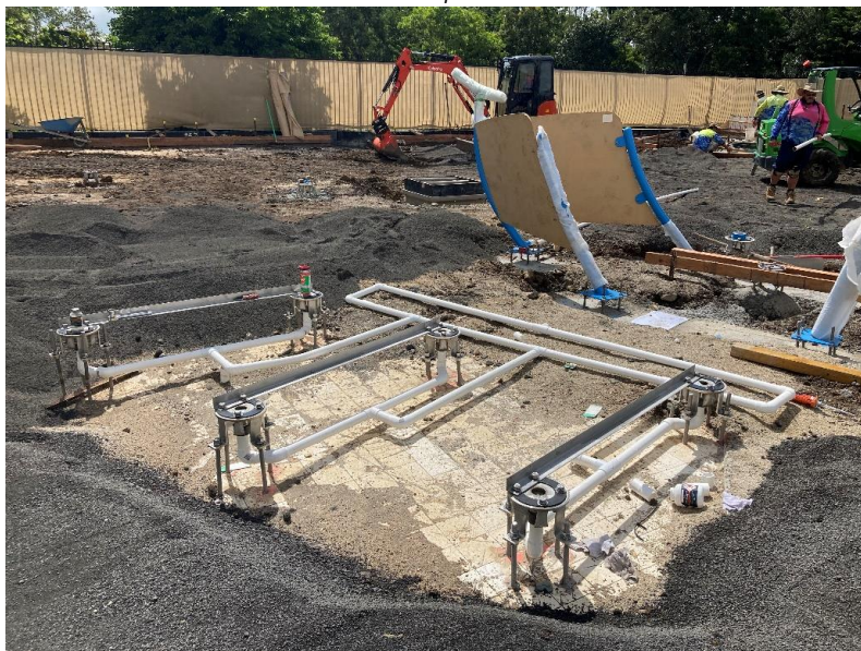
Plumbing and Play Equipment Preparation
