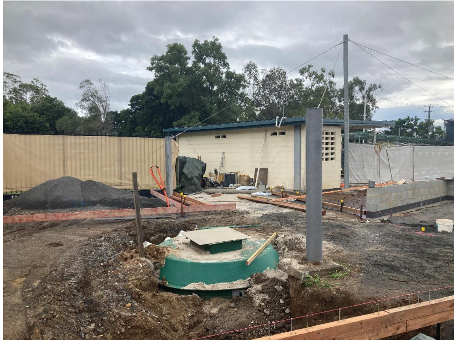
Installation of Balance Tank for Splash Park
