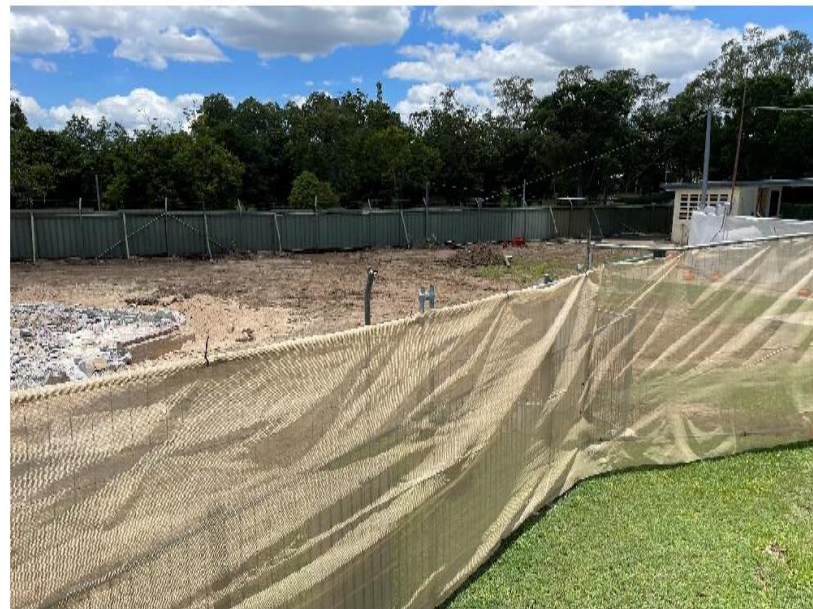
Site Clearing for Splash Park
