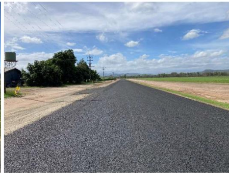
Borzi Road - After
