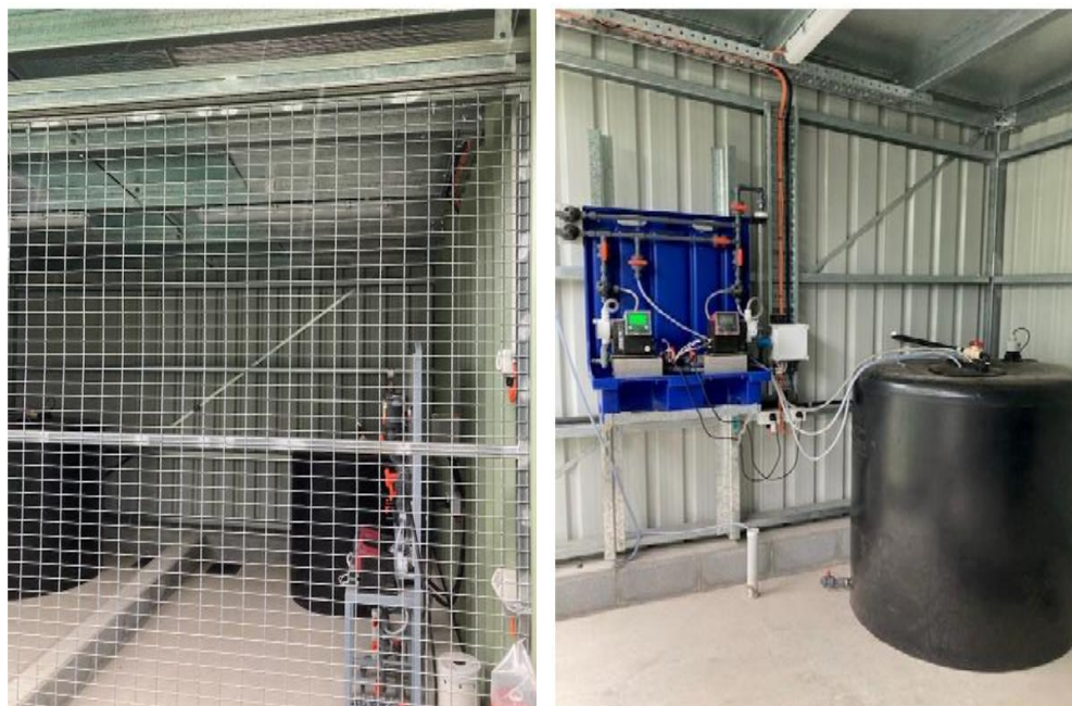
New chemical dosing shed and equipment
