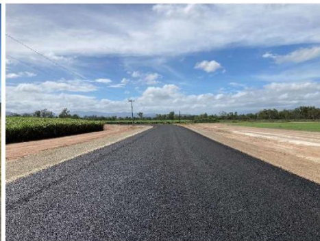
Borzi Road - After
