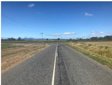
Borzi Road - Before
