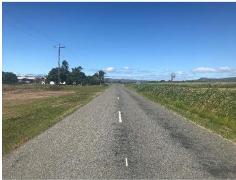
Borzi Road - Before
