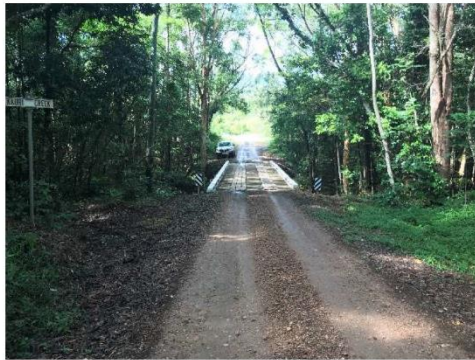
Kauri Creek Bridge - Before
