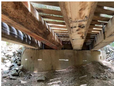
Newly installed girders
