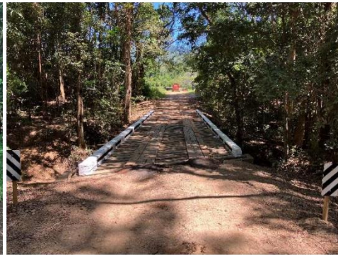
Kauri Creek Bridge - After
