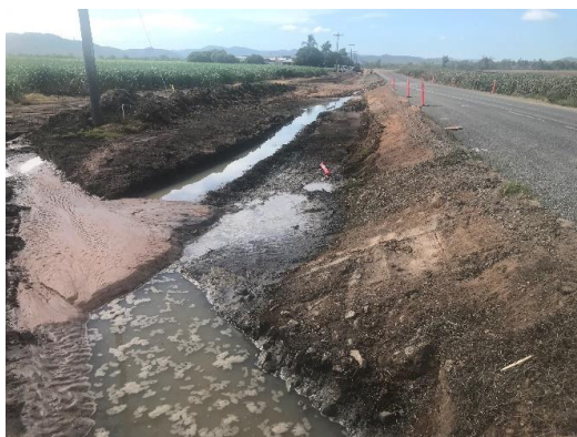
De-watering the site
