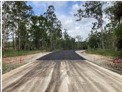
Completed first coat seal - Section A
