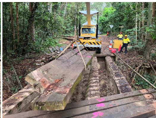
Bridge deck removal
