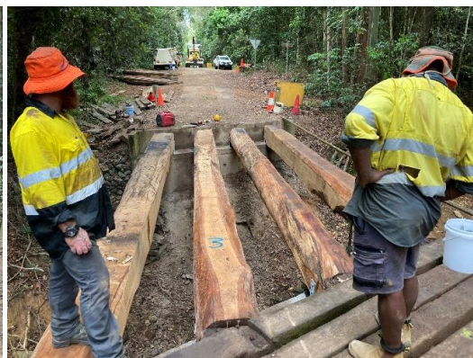
Replaced girders - span one
