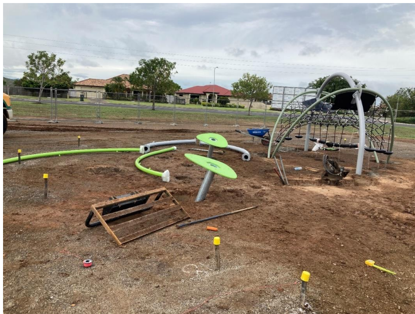
Photo 6 Mareeba East Park Play Elements Installation
