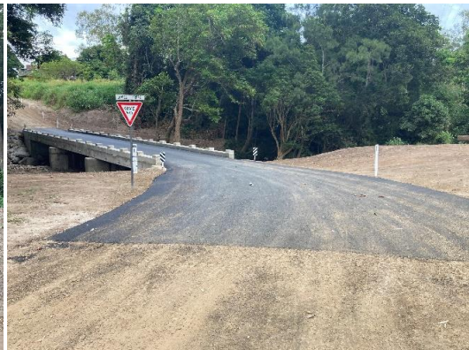
Eastern bridge approach
