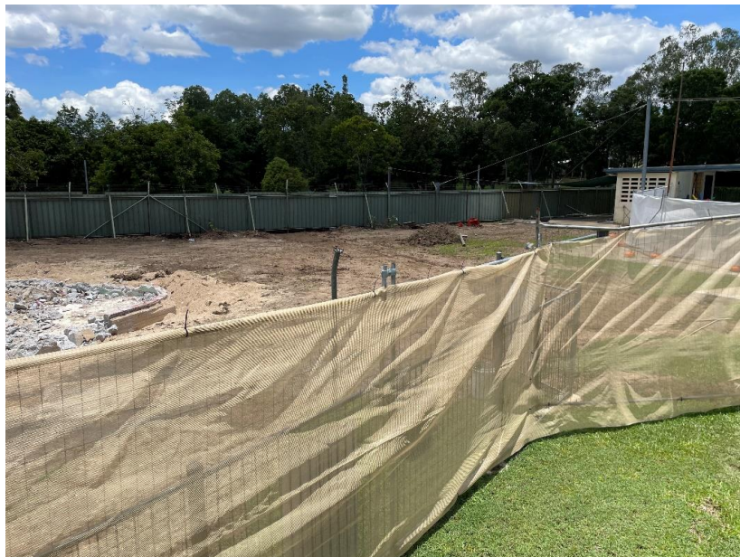
Photo 9 Site Clearing for Splash Park
