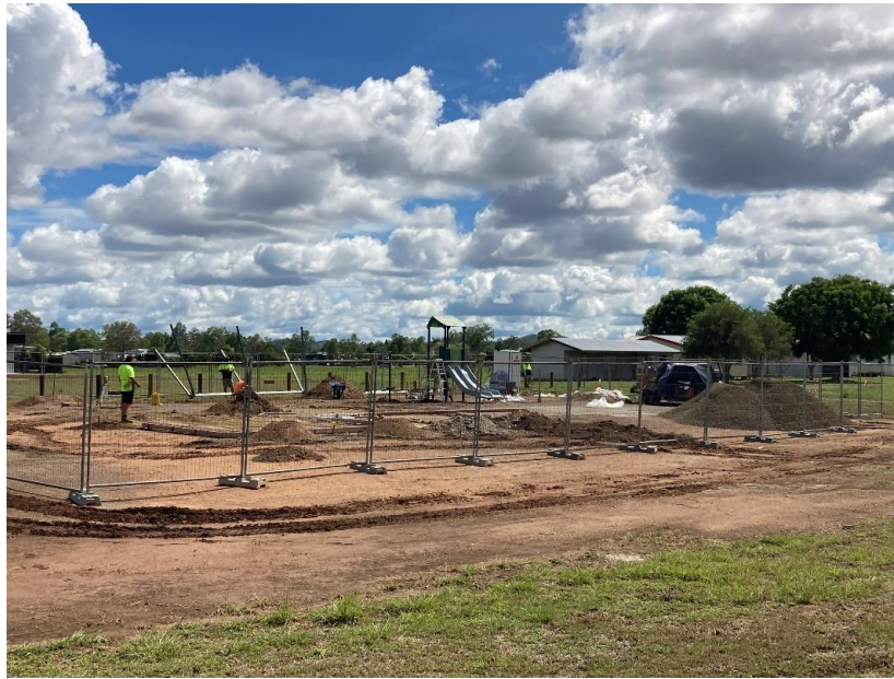
Photo 5 Mareeba East Park Playground Construction
