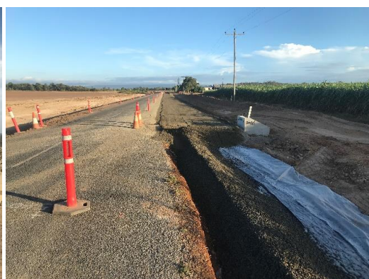
Installation of road base
