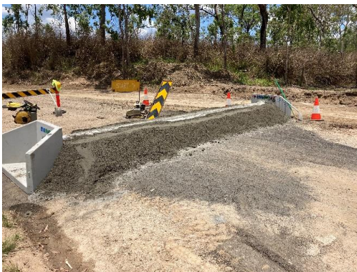
Hawkins Road RCP
