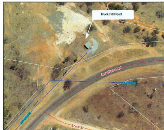
Frew Street/Aerodrome Road, Chillagoe
