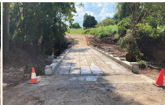
Completed concrete superstructure
