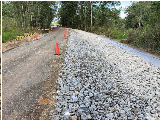
Completed rock mattress - Section B
