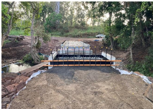
Western relieving slab formwork
