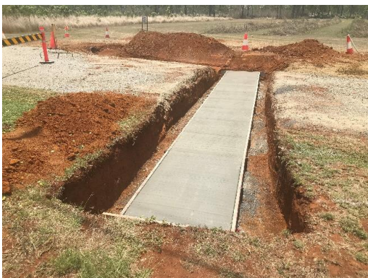
Mclver Road RCBC concrete base
