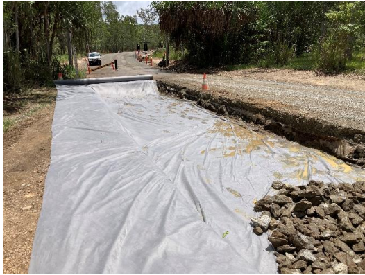
Replacement of unsuitable subgrade - Section B
