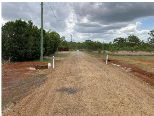
Mclver Road RCBC - complete
