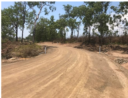
Hawkins Road RCP - completed
