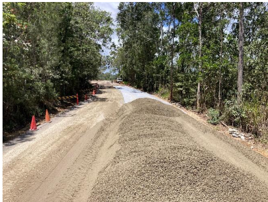
Importing road base - Section B
