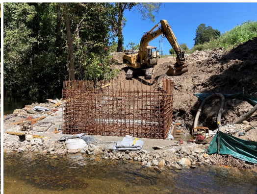
Steel reinforcing in place-western abutment
