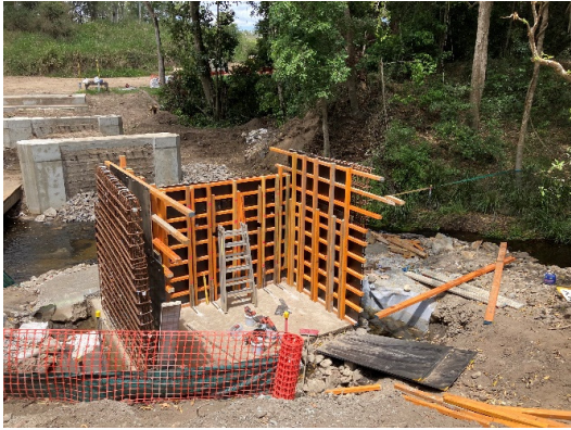
Commencing formwork-western abutment
