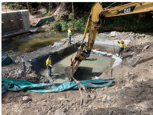
Pouring concrete blinding layer- western abutment
