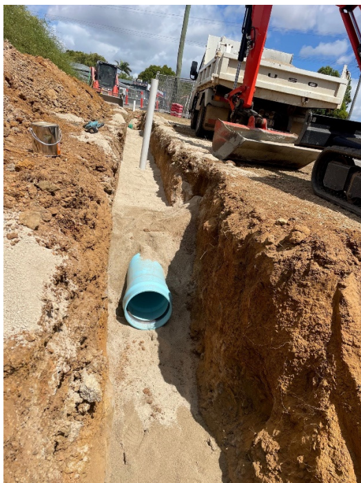
Herberton Street installation of the new 300mm diameter PVC Supermain water main
