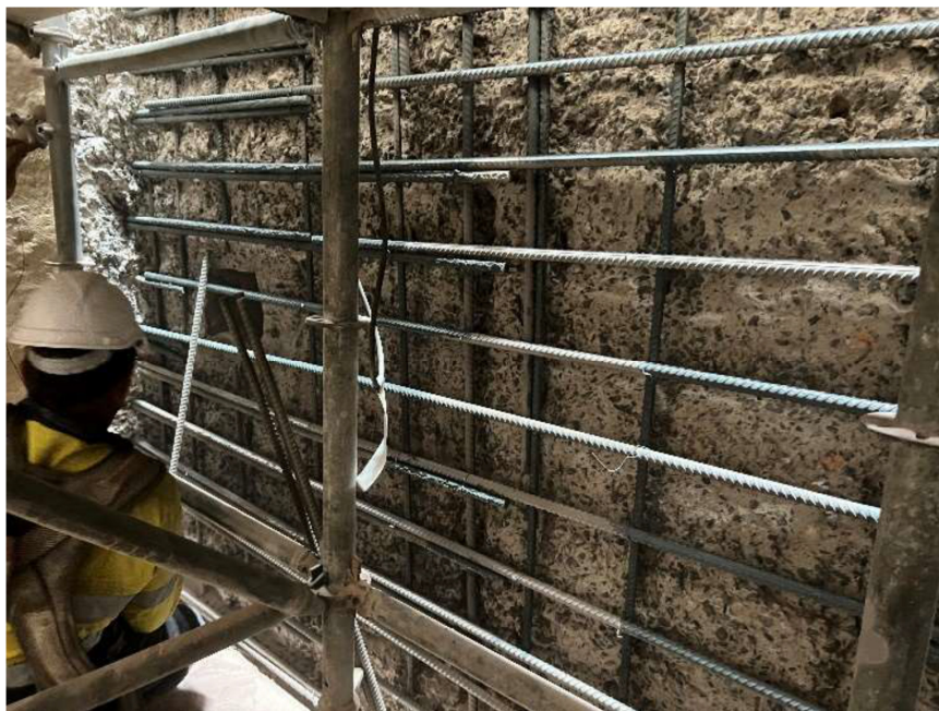
Divider wall remediation Granite Creek SPS
