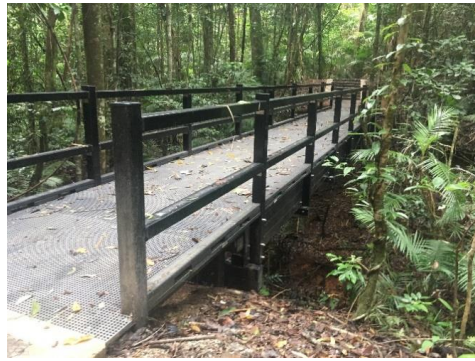
Bridge 6 National Park Section
