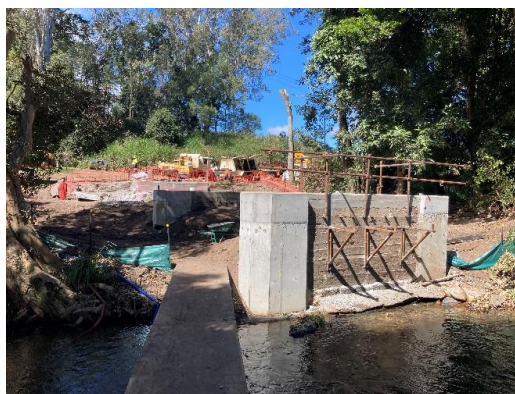
Completed pier extensions
