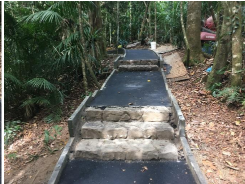
Jum Rum Trail - New pre-cast stone look concrete steps
