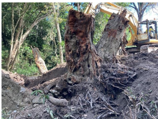
Removing western side tree stumps
