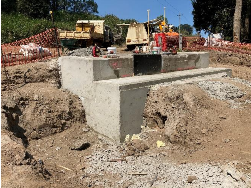
Completed east abutment & relieving slab
