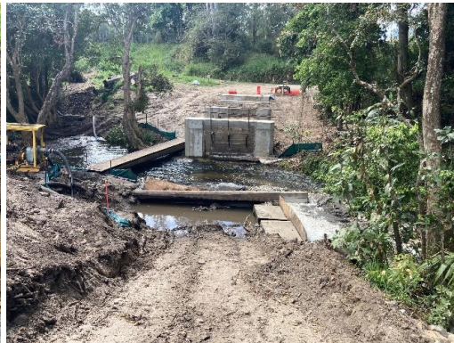
Dewatering west abutment excavation
