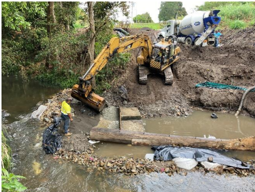
Pouring temporary concrete bund wall
