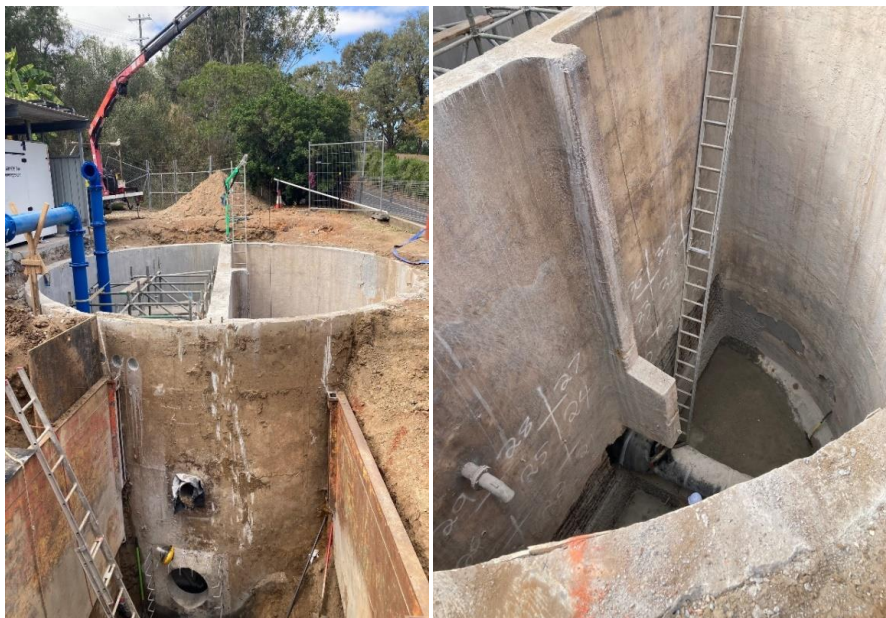
Excavation for new pipework and pipework intrusion, divider wall remediation Granite Creek SPS
