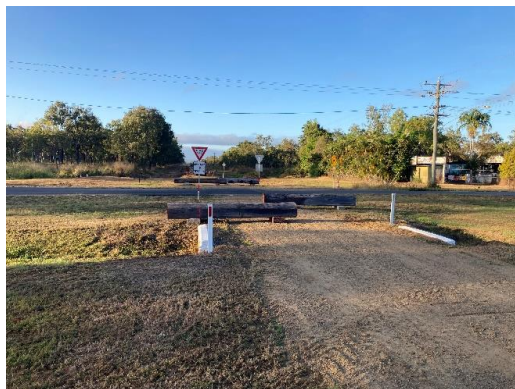
Signage and chicane arrangement
