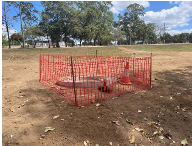
Installations of the new flow meter, pipe work to accommodate new bulk flow meter housed in concrete chamber opposite the Mulligan Highway near Granite Creek
