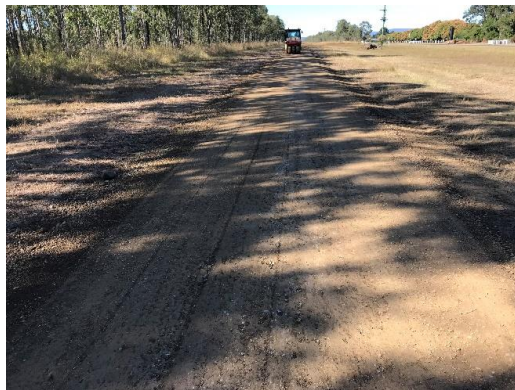
Static rolling of the trail
