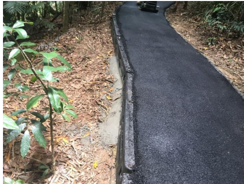
Jum Rum Trail - Asphalt overlay and buttressed edge
