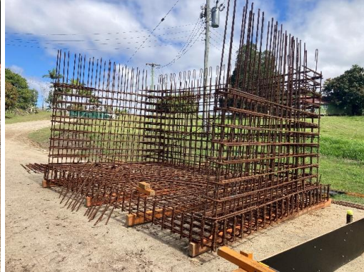
Western abutment reinforcing
