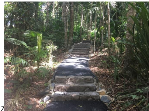
Jungle Trail - Replacement stone look steps
