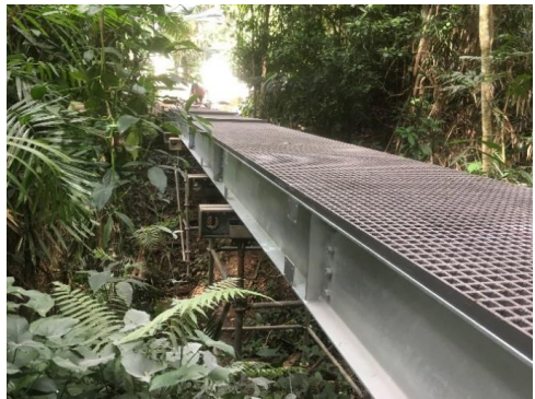
New Barang Street Bridge - Under construction
