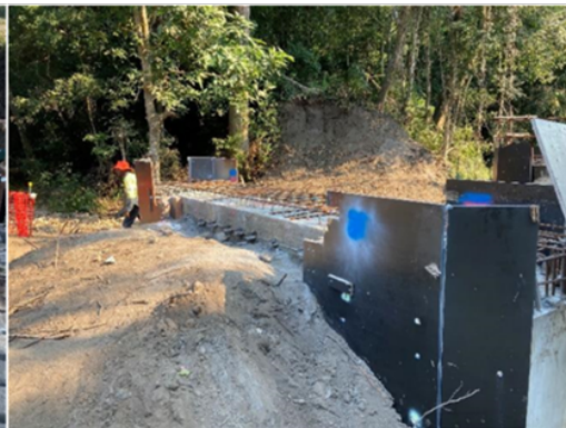
Completed pier extension steel and form work
