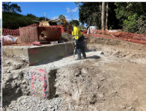
Preparations for abutment renewal
