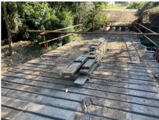
Demolishing existing timber bridge deck
