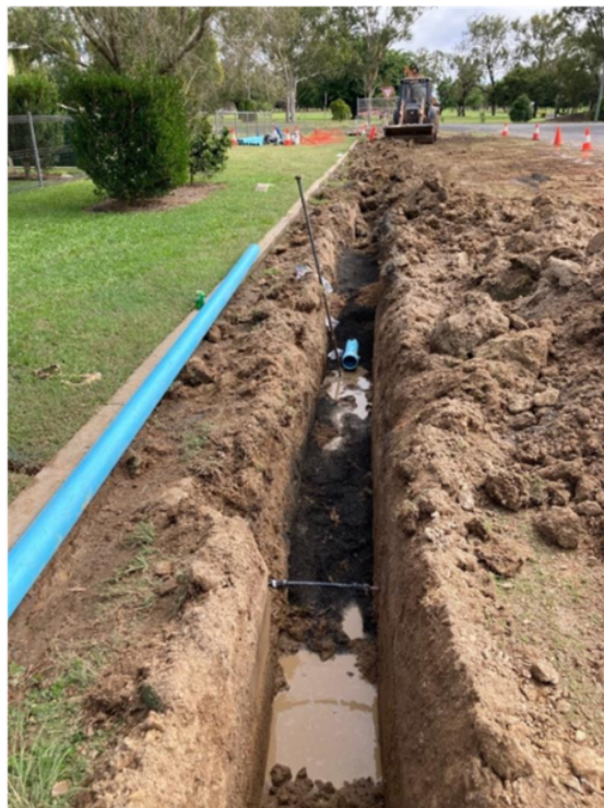
Rice Street installation of the new 100mm diameter PVC Supermain water main
