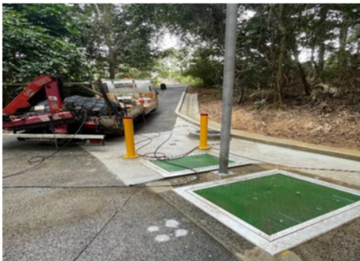
Thooree Street – Kuranda • Project completed
