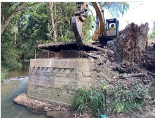
Removal of existing relieving slabs
