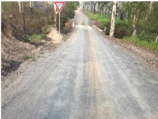
Davies Creek Road bridge (before)
