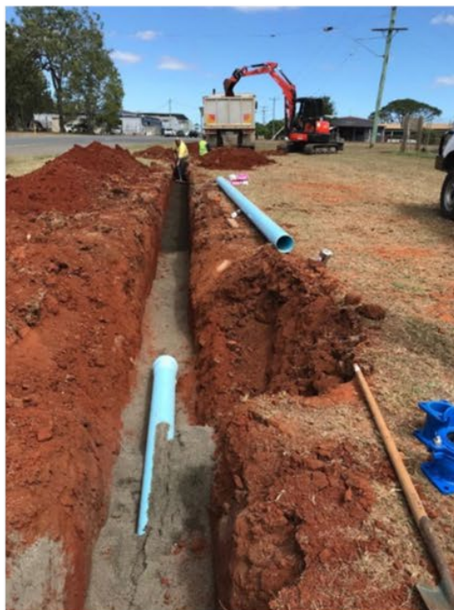
Chewko Rd onto Hales St installation of the new 150mm diameter PVC Supermain water main
