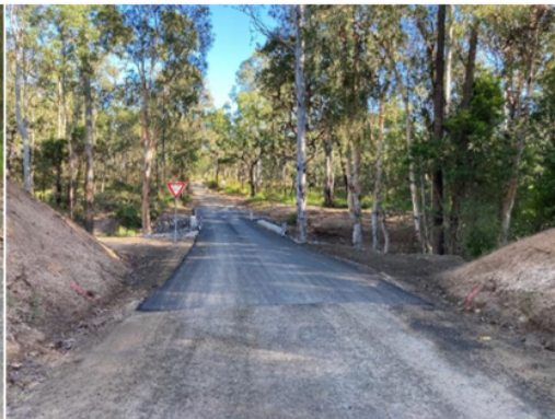
Davies Creek Road bridge (after)
