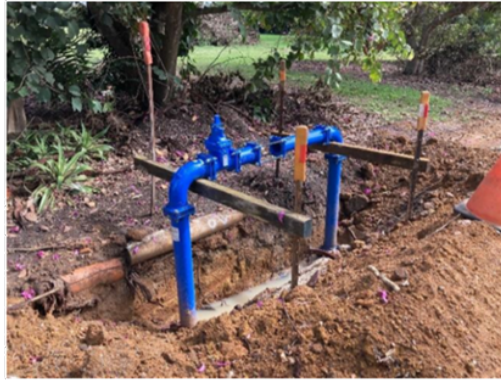
Installations of the new pipe work to accommodate new flow meter to Baiada (Steggles) on Moody Street
