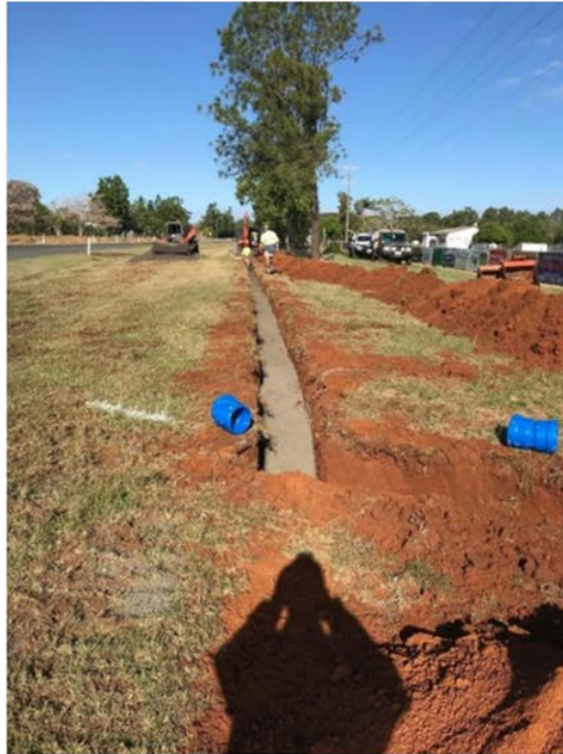
Chewko Rd installation of the new 150mm diameter PVC Supermain water main
