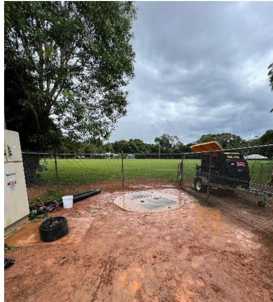
Works completed at Arara Street, Kuranda
