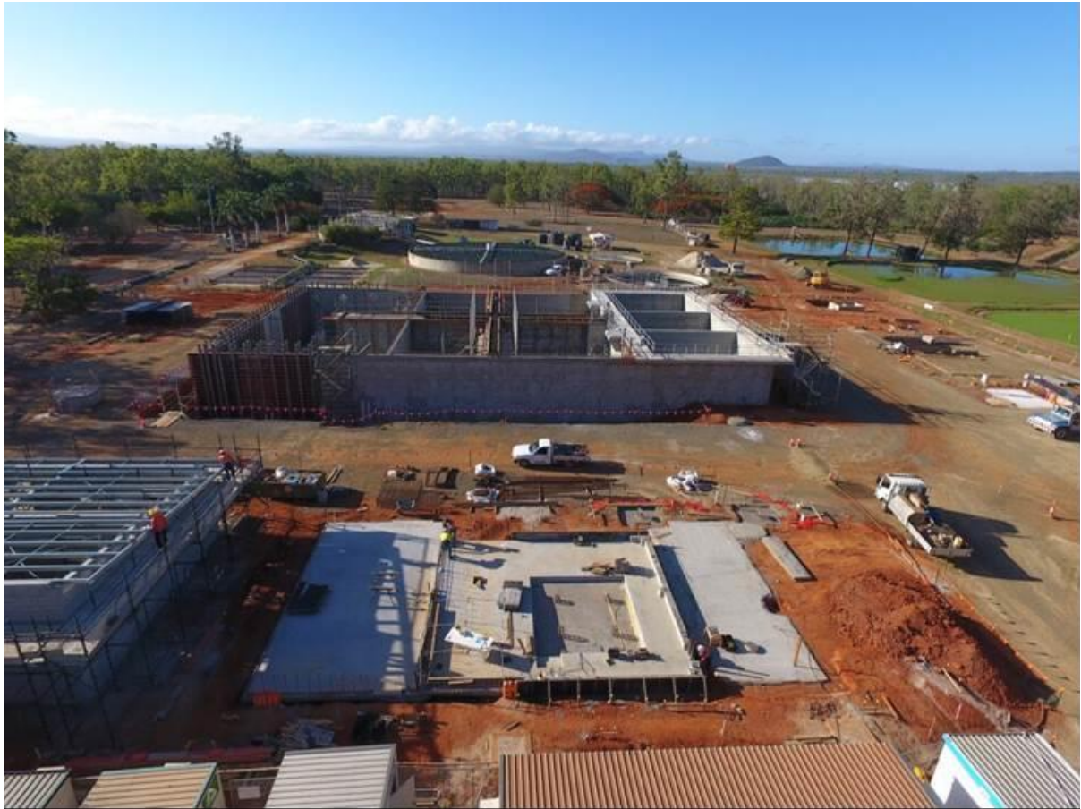
20 December 2016 - Roof installation to the Admin and MCC Building and the slab has been completed for the blower building and biosolids dewatering building.
