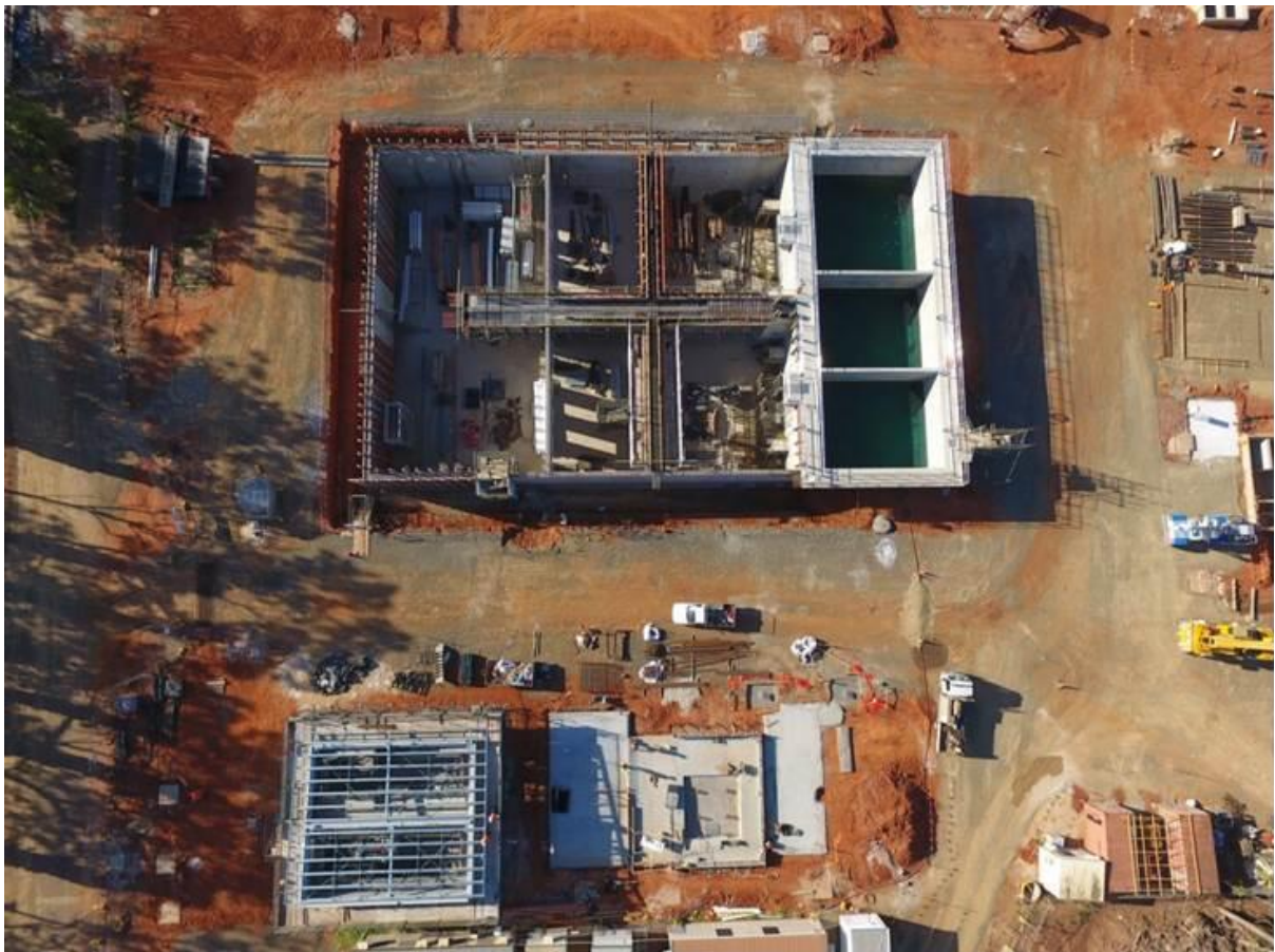
20 December 2016 - Filling of the digester cells in the SBR structure with water for hydrostatic testing
