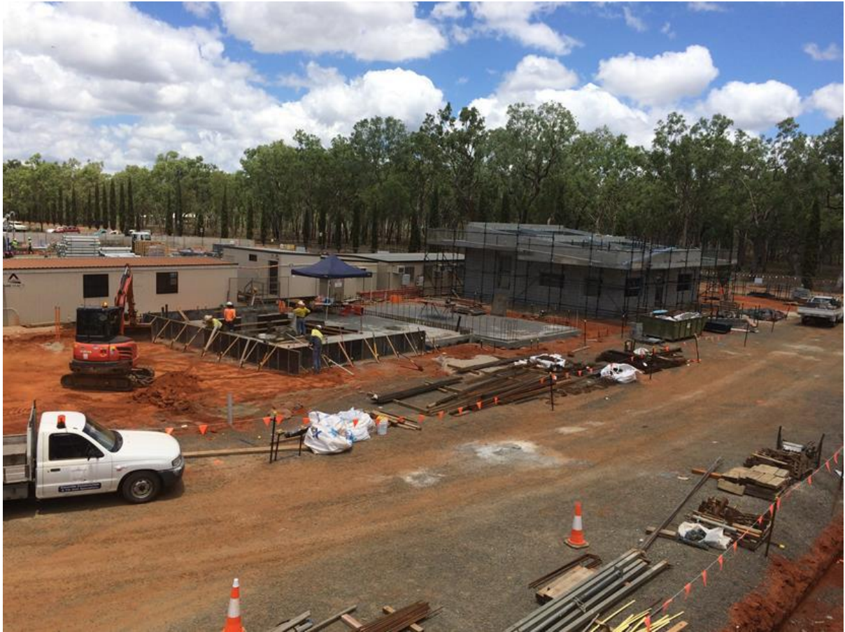
15 December 2016 - Roof installation to the Admin and MCC Building and concrete slab construction for the biosolids dewatering building.
