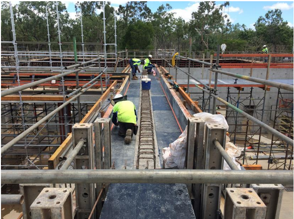
15 December 2016 - Construction of elevated walkways to sequential batch reactor (SBR) structure.
