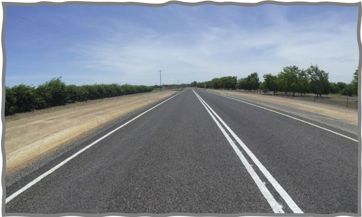
Photo 5 Dimbulah Leedingham Creek Road CH1.65-2.57
