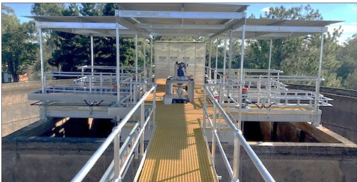
Photo 3 Mareeba WTP Clarifier Refurbishment
