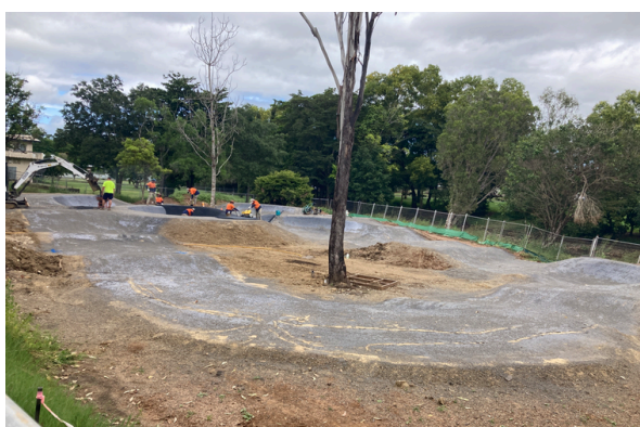
Pump Track Installation
