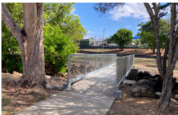
Keeble Street Footbridge Restoration
