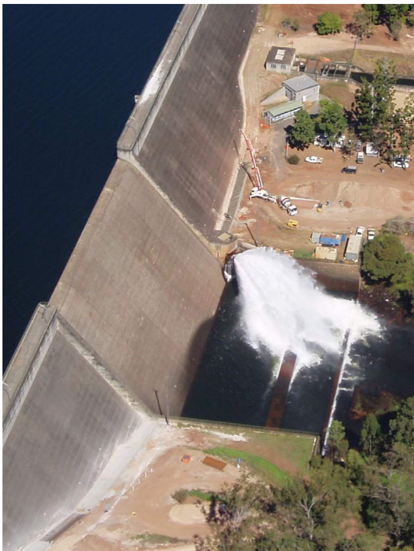
'Tinaroo Dam Wall', Photo courtesy: Cassie McLucas
