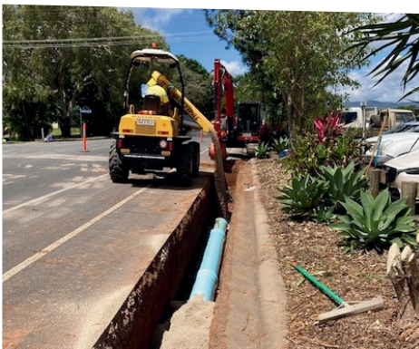
AC water main replacement program
