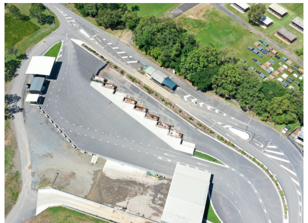
Mareeba Transfer Station Redevelopment, 2021
