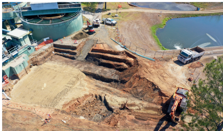
Mareeba Water Treatment Plant filtration system upgrade
