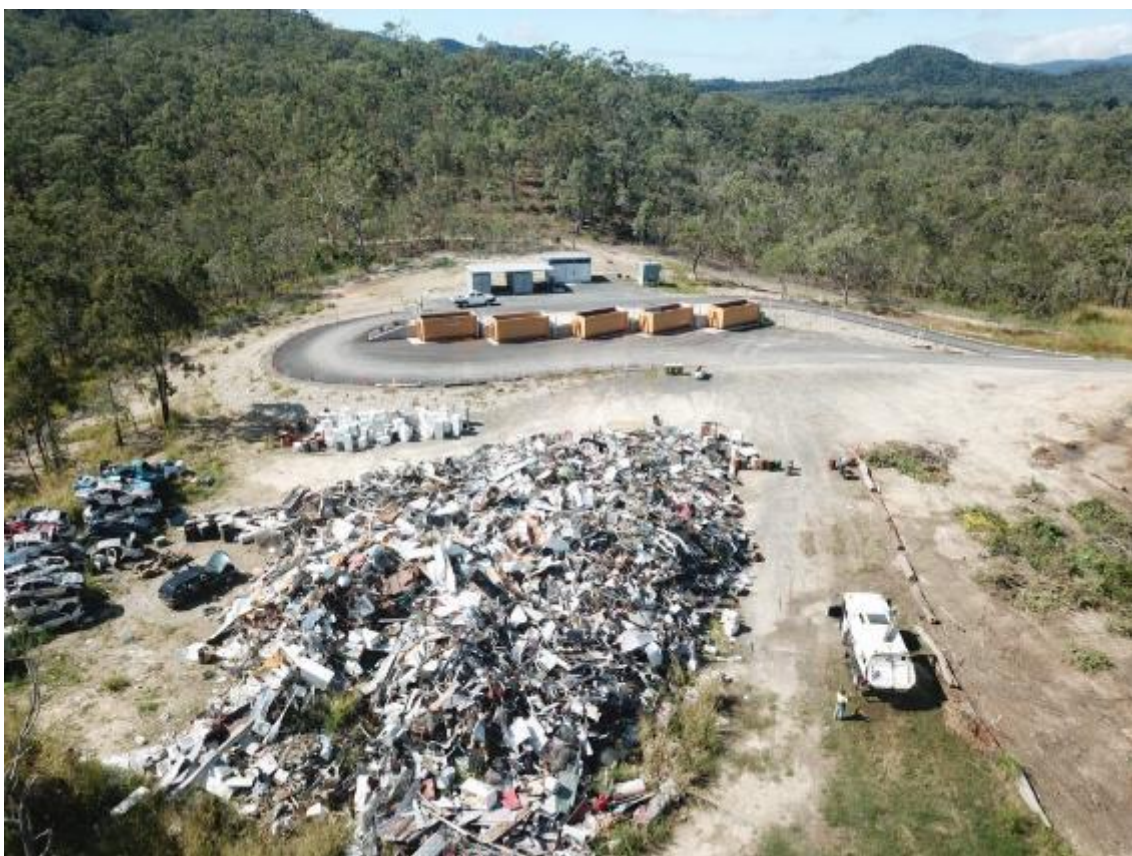
Figure 15 Upgraded Kuranda Waste Transfer Station 2017
